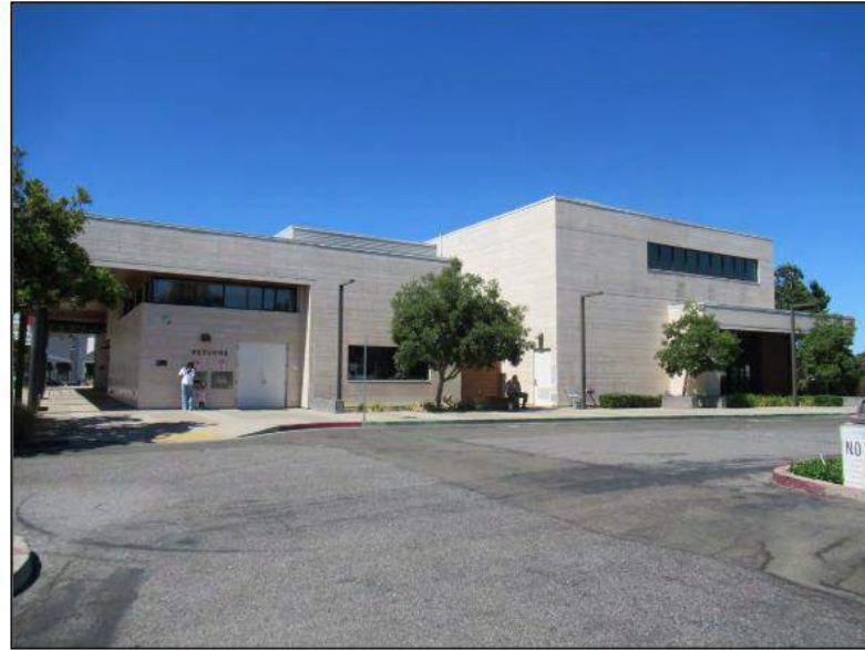
43. East elevation as seen from the parking area.
