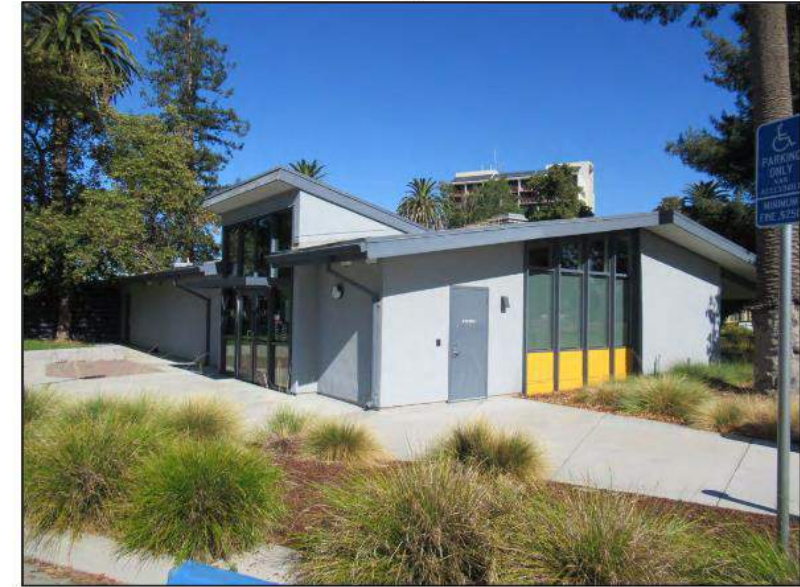
31. East and south elevations looking north.
