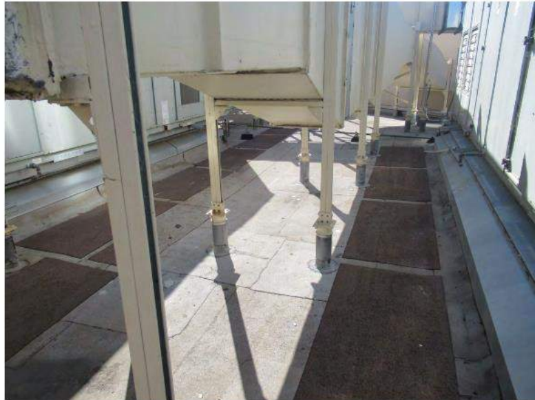
24. Roof membrane and walking pads at the RTUs.
