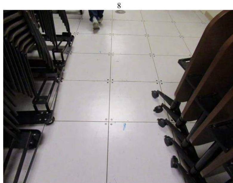
8. Typical raised floor throughout the facility.
