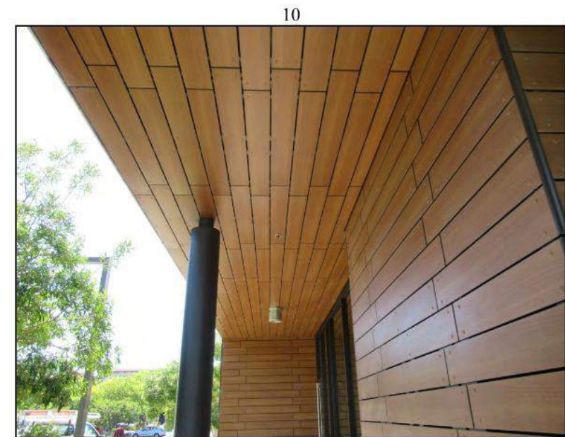
10. Soffit and wall rainscreen cladding is faux wood panels.
