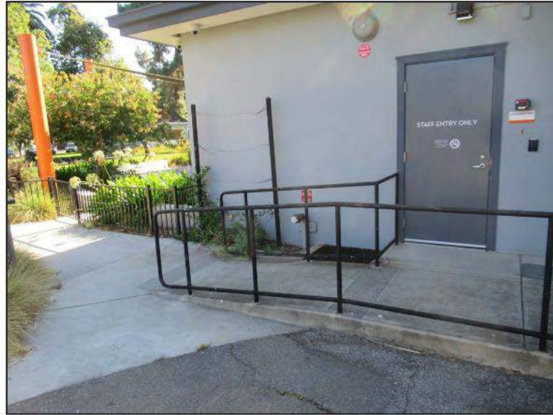
9. South side of building with employee access.
