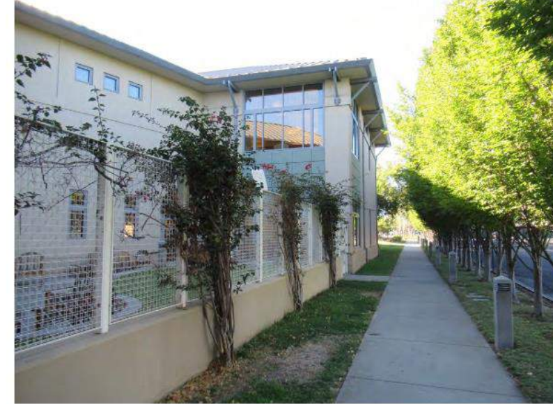
21. View of the west side of the building.
