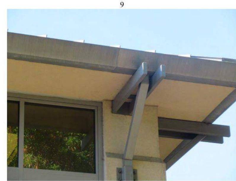
9. View of the eave, soffit, copper gutter and downspout.
