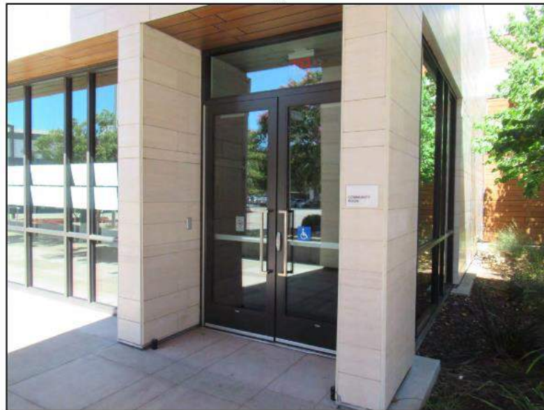
40. Pedestrian entrance to the community rooms.
