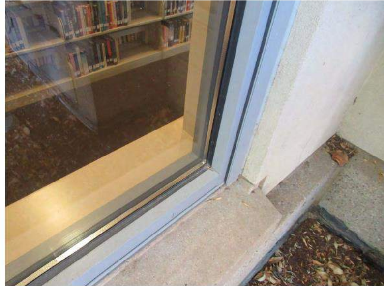
11. Windows are aluminum frame with insulated glazing.
