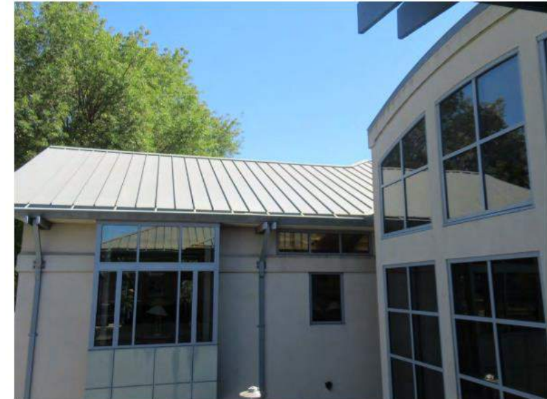
26. Typical standing metal seam roof membrane at the sloped roofs.
