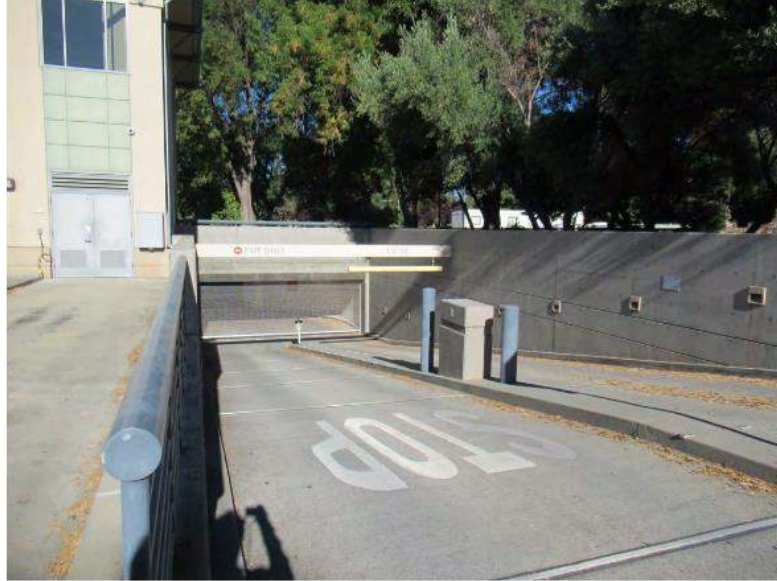
19. Entry to the garage is on the northeast corner of the building.
