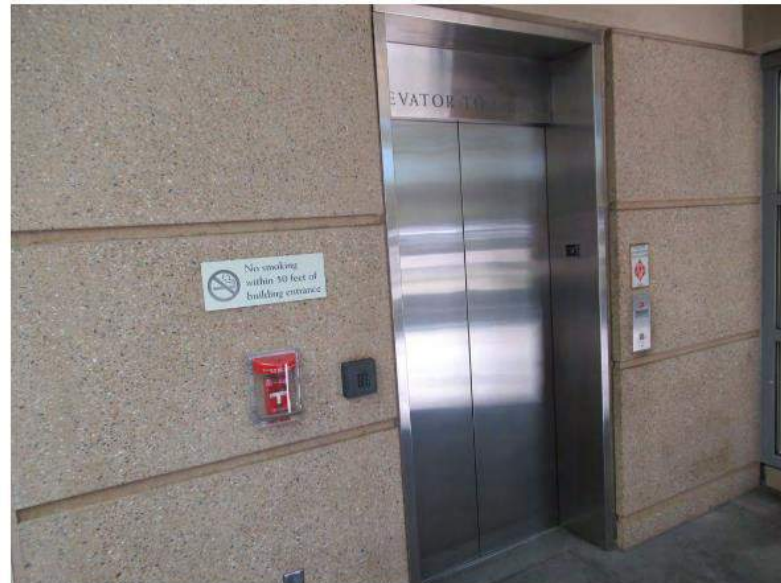
52. Exterior passenger elevator serves the ground floor and garage levels.
