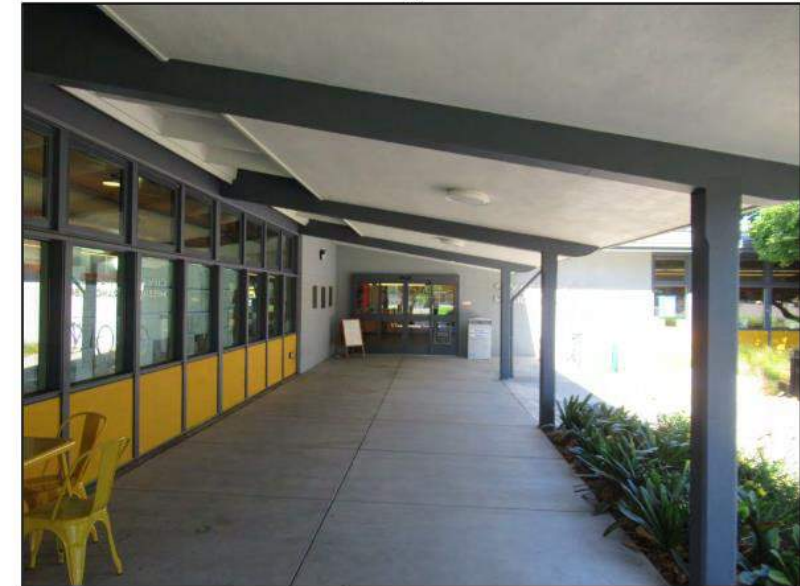
12. Colonnade leading to the main pedestrian entrance.
