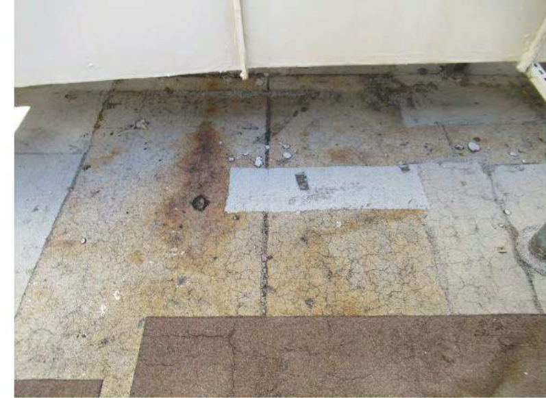
25. Condition of the roof membrane is considered fair.
