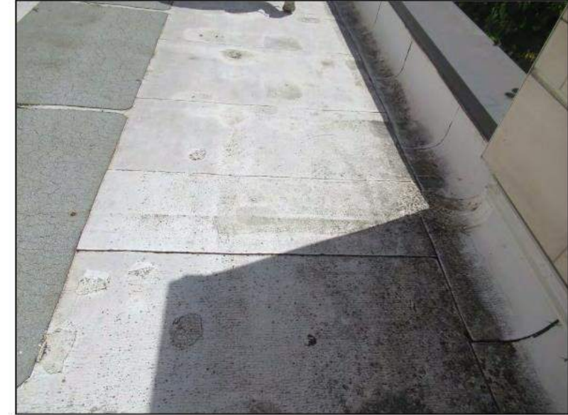
17. Membrane appears to be a multiply torch down system.
