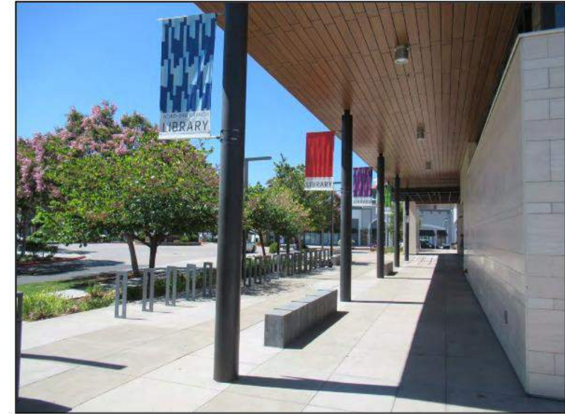
41. Colonnade along the south side of the building.
