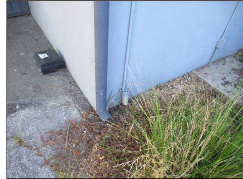
7. Downspouts discharge at grade.
