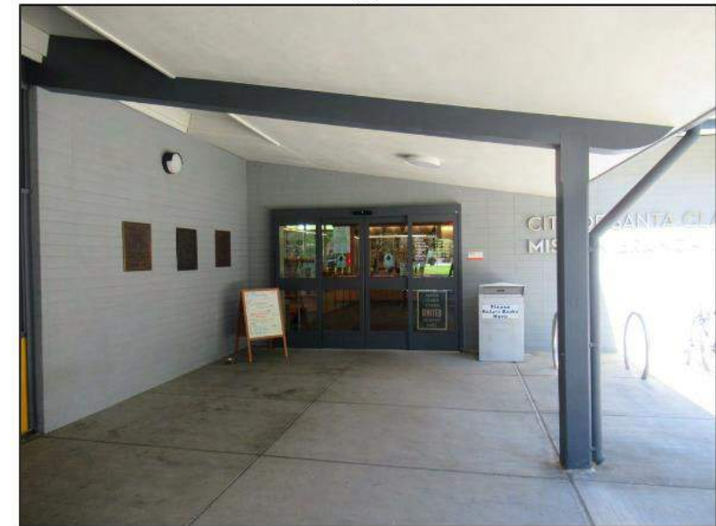
32. Main pedestrian entrance, east side of the building.
