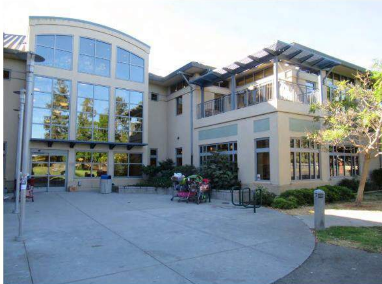
20. View of the west side of the building.
