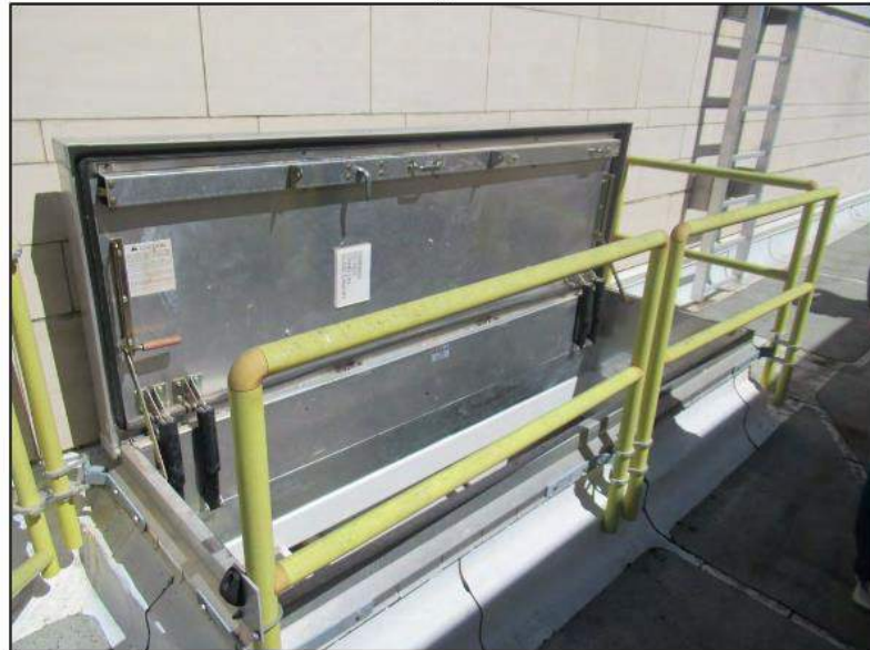
16. Roof hatch accessed by stairs off the lobby.
