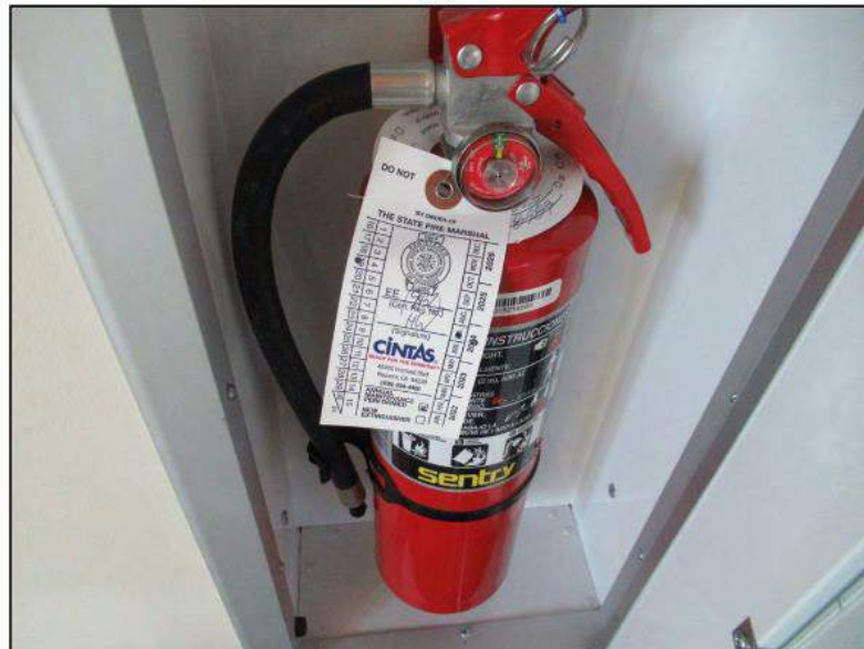
26. Fire extinguishers have current service tags.
