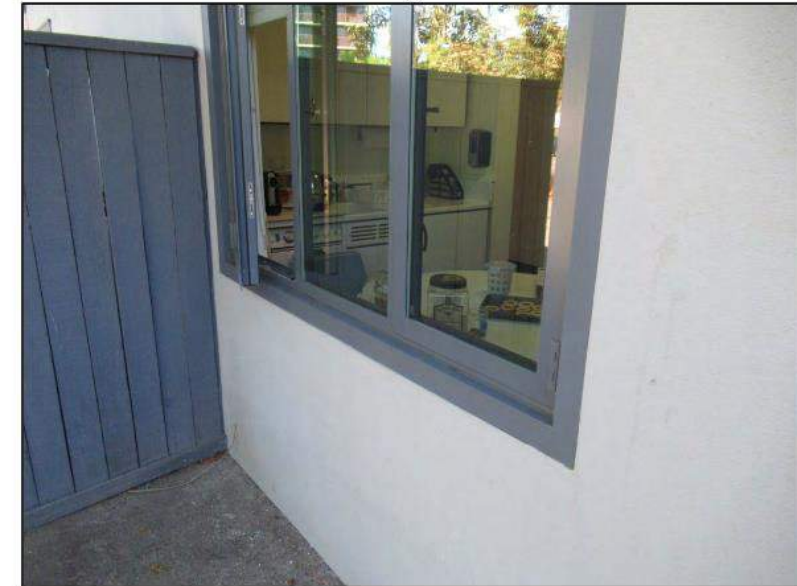
8. Typical aluminum framed casement windows with insulated glazing.
