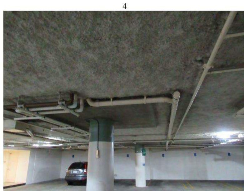
4. Ceiling of the garage has a fire proofing.
