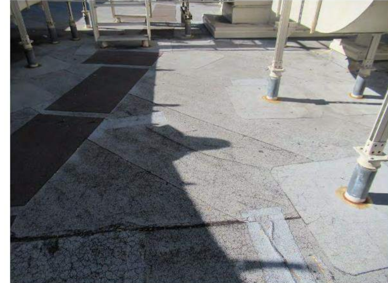
22. Membrane is original installed in 2004.
