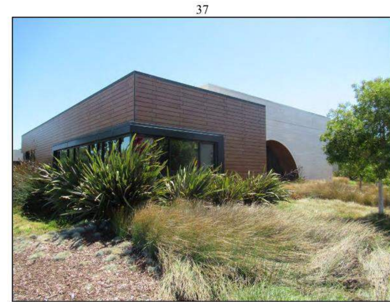
37. Northwest corner of the building as seen from the park.
