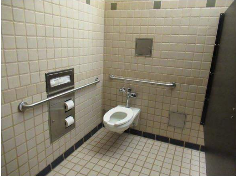
42. Toilets have automatic flush valves.
