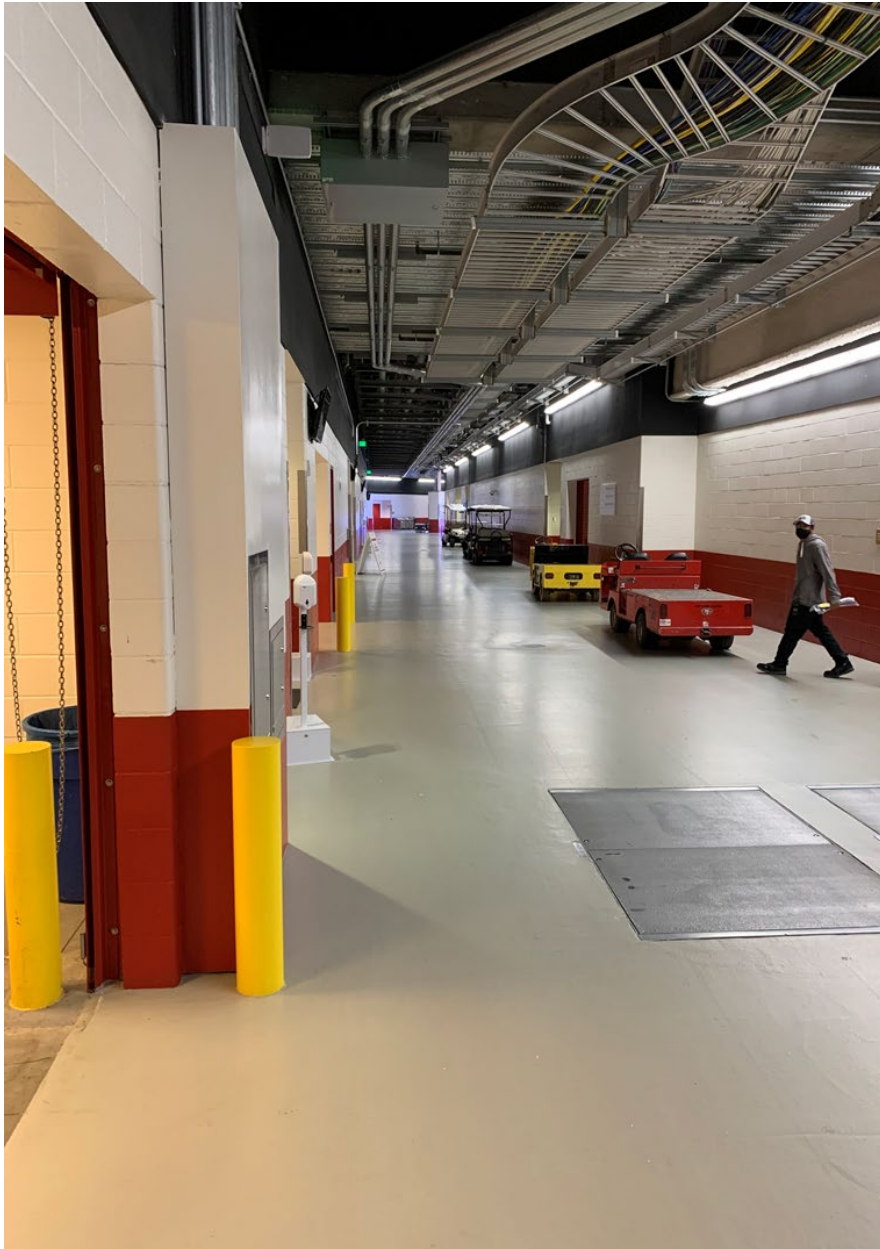
Figure 5: Photo of Corridor to Auxiliary Rooms (ALTERNATE #1 BID SCOPE) look into corridor tunnel area from field area.
