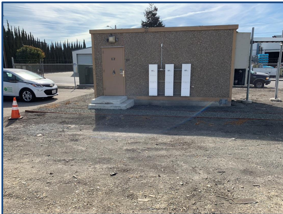
View of the existing electrical shed structure on the subject
