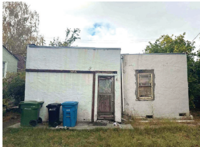
Photograph 4: 520 Hilmar St, southeast elevation, camera facing northwest, November 13, 2024.
