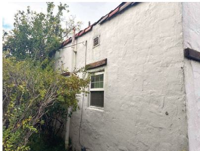
Photograph 5: 520 Hilmar St, southwest elevation, camera facing northeast, November 13, 2024.
