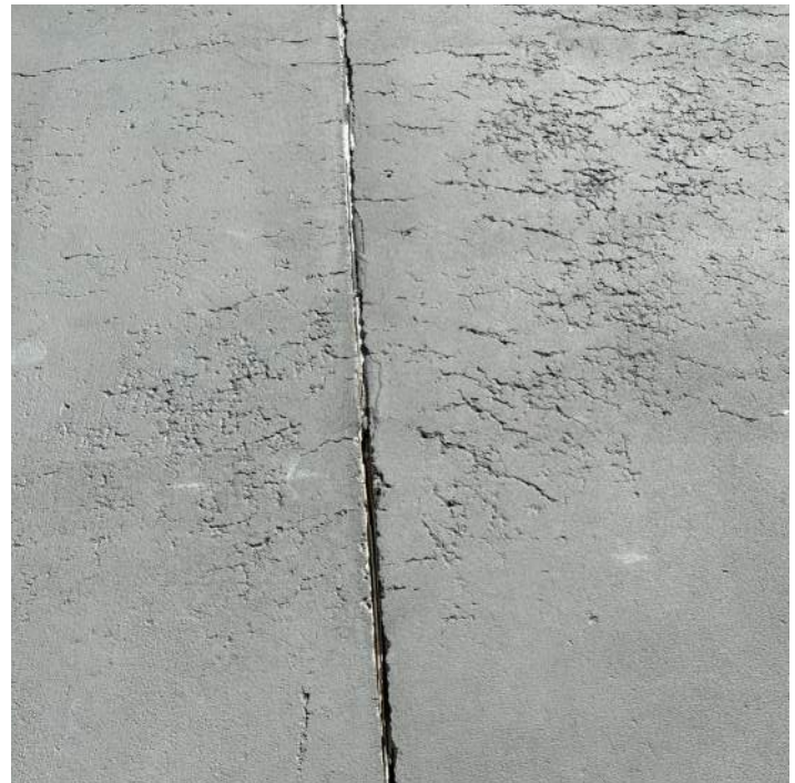
Image 18: Failing Pool Deck
