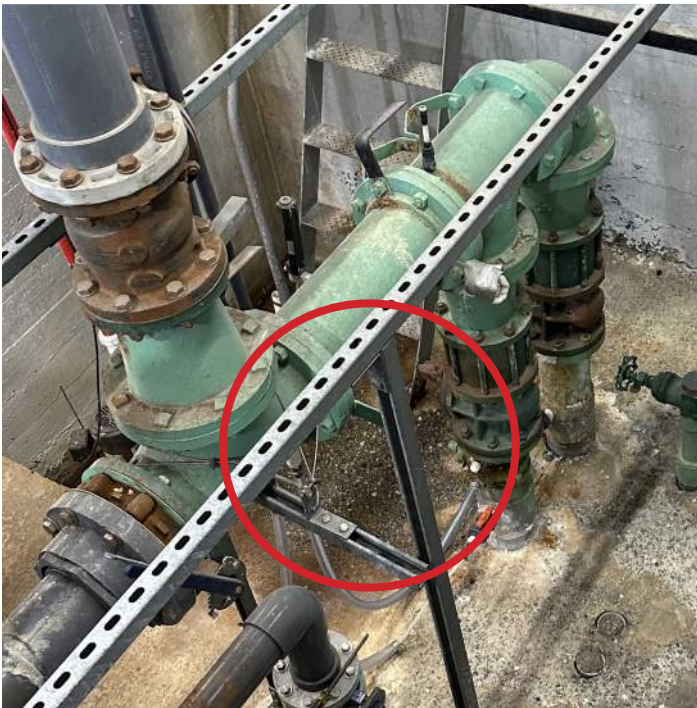
Image 21: Evidence of Leak in Pump Pit
