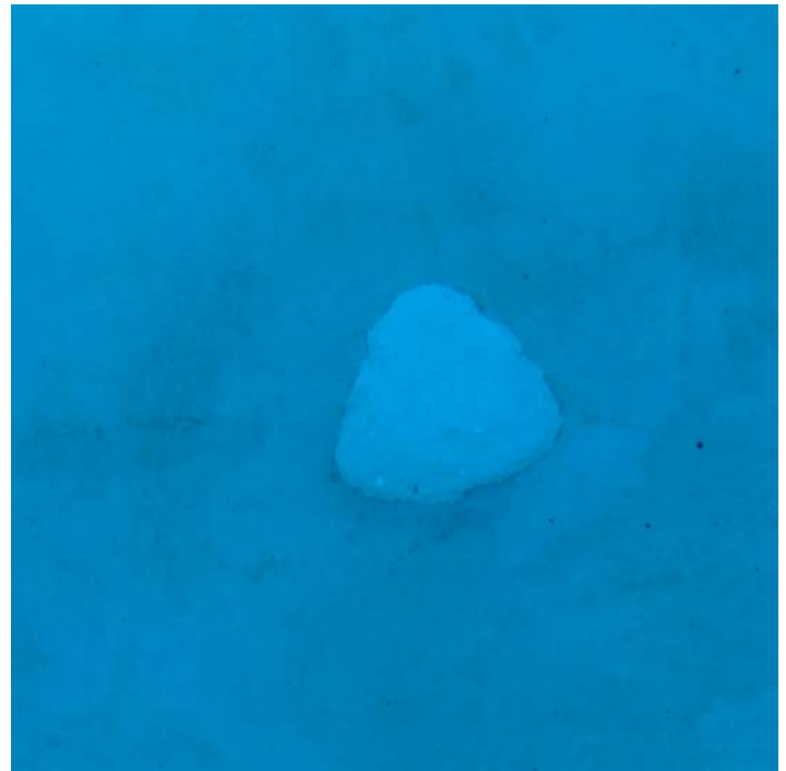
Image 16: Delaminating Plaster in Diving Pool
