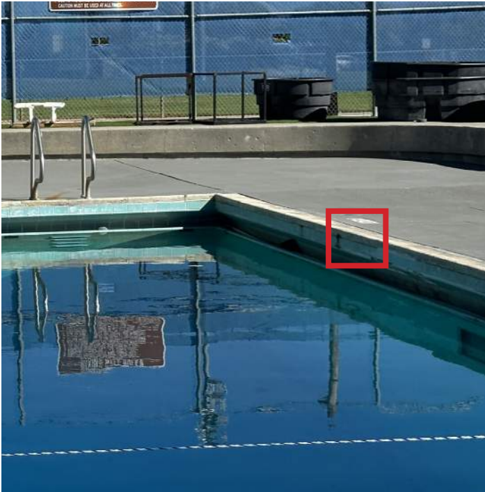
Image 19: No Waterline Depth Marker
