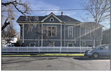
EXISTING PHOTO #P2
