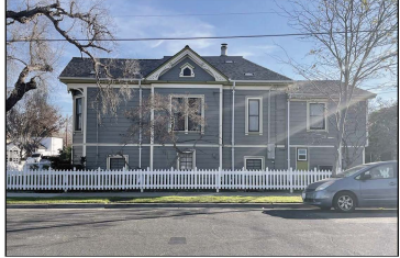
EXISTING PHOTO #P2
