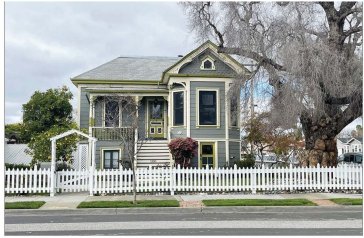
EXISTING PHOTO #P1
