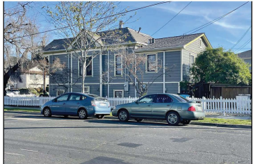
EXISTING PHOTO #P3
