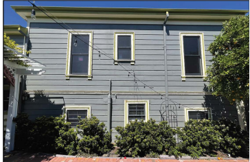
EXISTING PHOTO #P4
