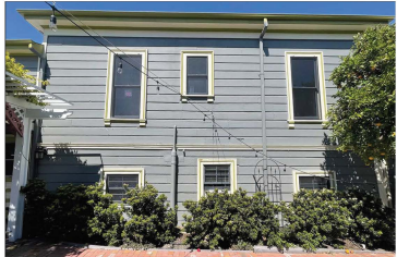
EXISTING PHOTO #P4
