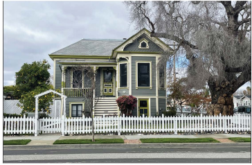
EXISTING PHOTO #P1
