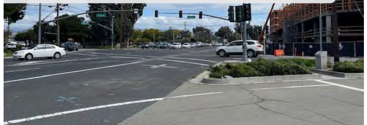
Project team investigates infrastructure on El Camino Real adjacent
