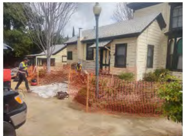
Repairs to Harris Lass
