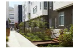
LINEAR STORMWATER TREATMENT @ CIVIC CENTER DRIVE FRONTAGE
