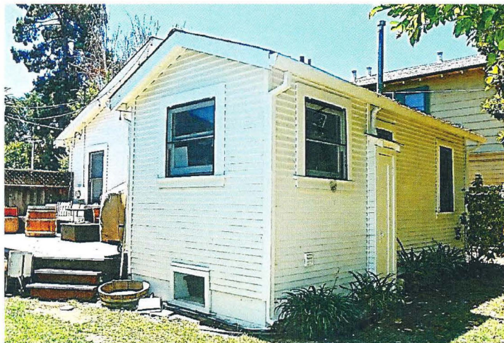
Photo No: 100_3074 View: Rear façade & E side-elevation of wing and deck with steps; Photo Date: August 2022; Camera Facing: S
