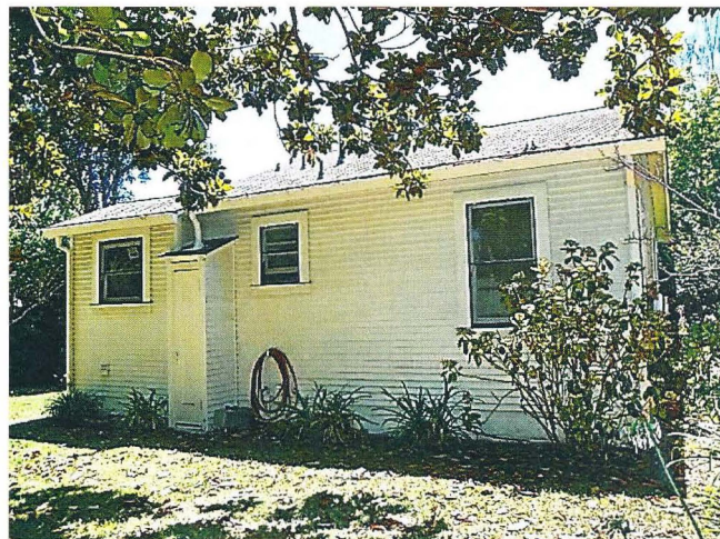
Photo No: 100_3080 View: Rear façade & partial W side-elevation. Photo Date: August 2022; Camera Facing: SE
