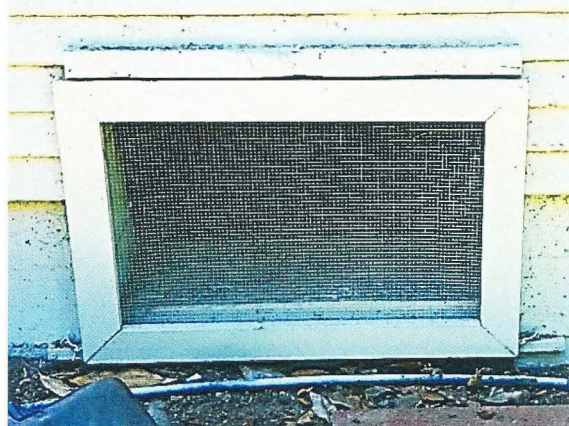
Photo No: 100_3092 View: Wood-framed crawl space vent with metal screen; Photo Date: August, 2022; Camera Facing: WSW
