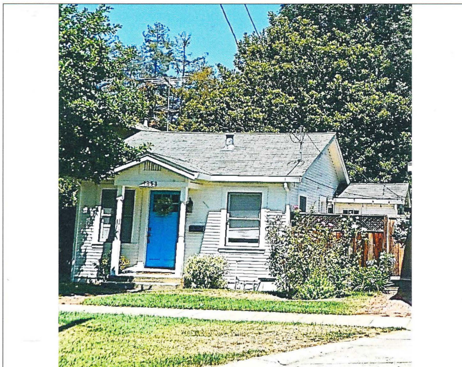
Photo No: 100-3055; View: Front facade & Partial E side-elevation showing wing; Photo Date: August 2022; Camera Facing: NW
