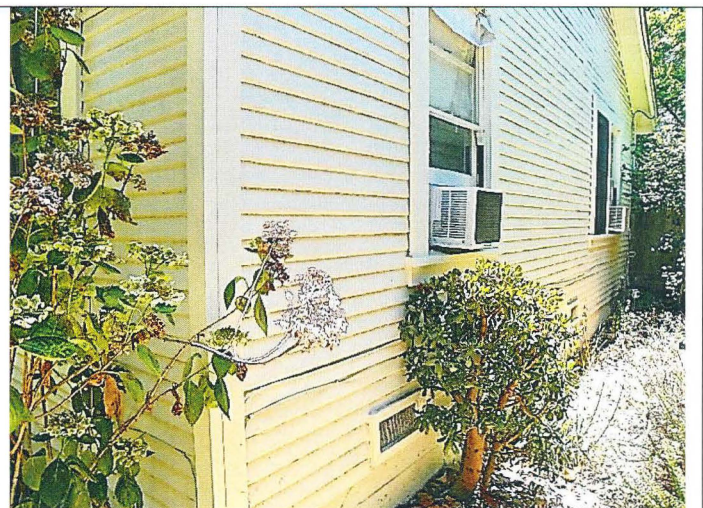
Photo No: 100-3083; View: Partial W side-elevation (bottom ½); Photo Date: August 2022; Camera Facing: E
