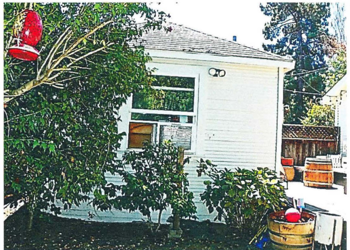
Photo No: 100_3071 View: Rear façade detached garage; Photo Date: August, 2022; Camera Facing: SSE
