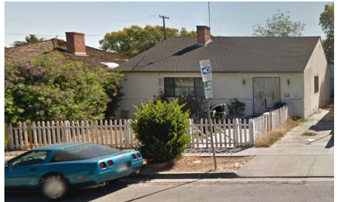
Figure 20. 970 Poplar Street, front elevation, October 2014 (Source: Google Street View).
