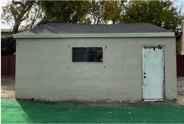
Figure 9. Garage, east (side) elevation.
