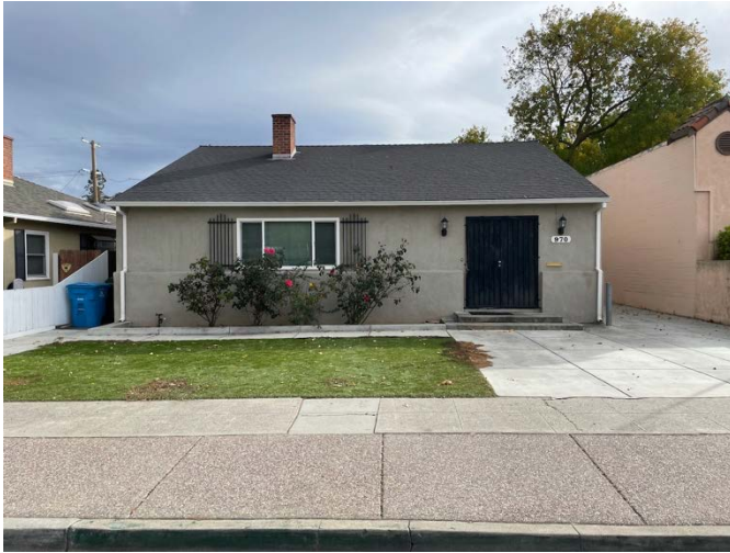
Figure 1. North (front) elevation with metal screen doors locked.
