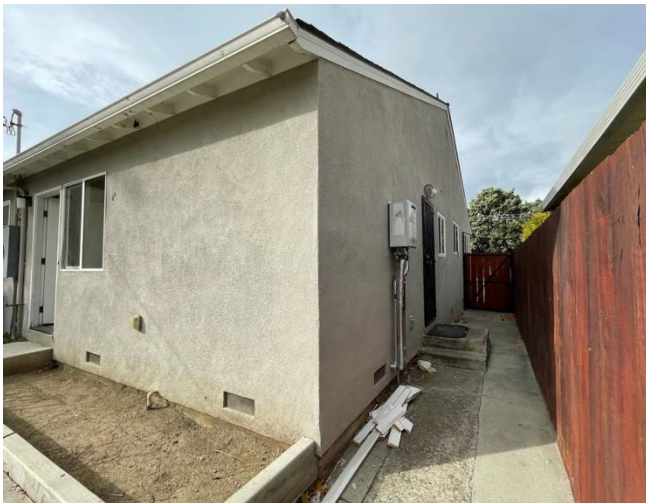
Figure 7. East (side) elevation, viewed from backyard.
