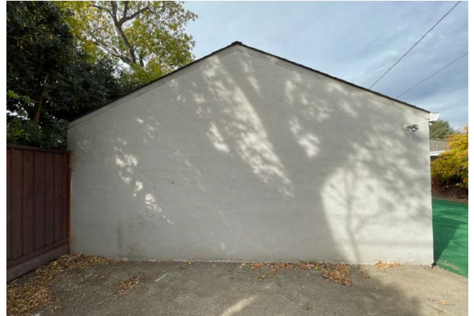
Figure 10. Garage, rear elevation.
