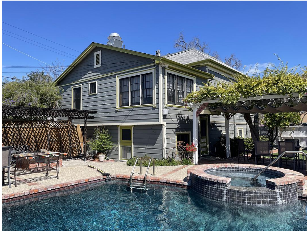
Figure 3: Rear addition built in 1972.
