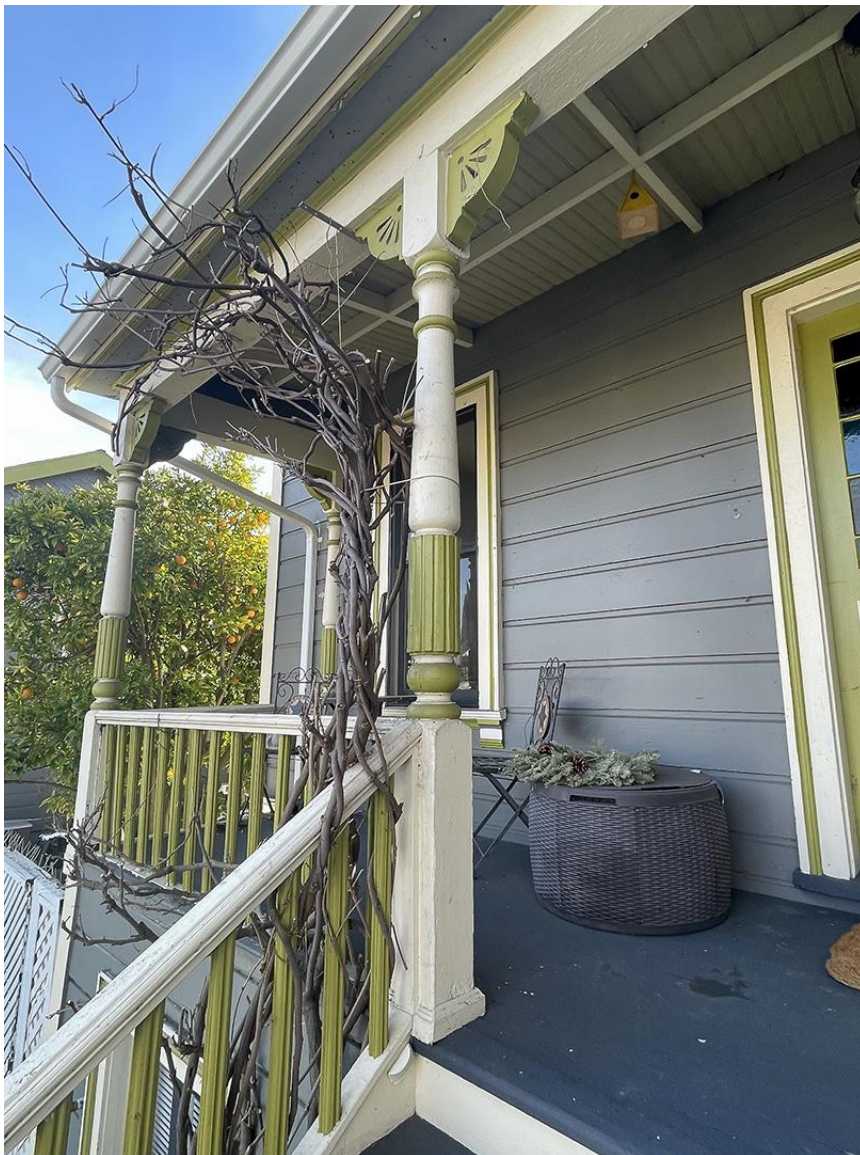
Figure 1: View of front porch with Victorian details.
