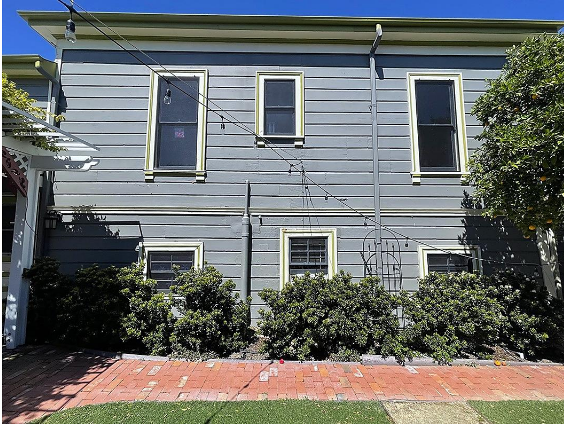
Figure 6: View of south elevation with non-historic windows on the basement level.
