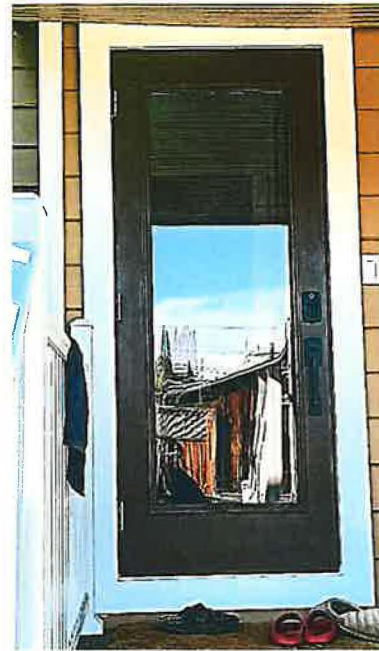
Photo No: IMG_1425; View: Rear Entry Door; Photo Date: 2/6/2026.
