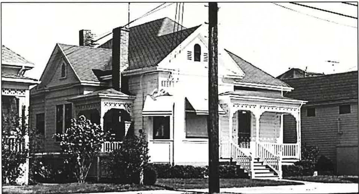
1261 Jackson Street (June 1980 Photo - note the window's projecting sills and aprons & missing side porch steps.)
