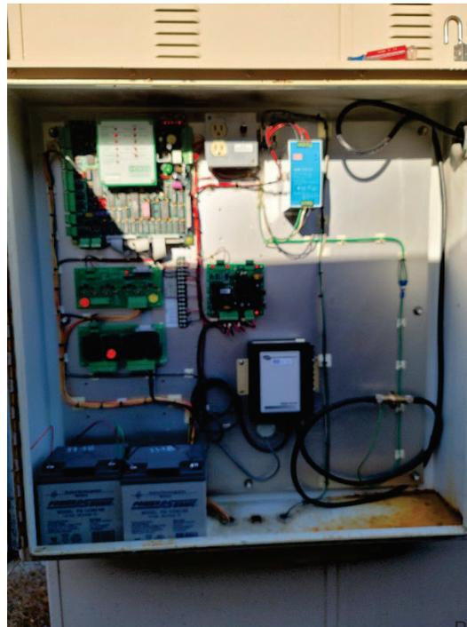
HSQ shall develop and design the two required RTU Back panels to retrofit to existing site enclosure and existing signals. Existing wiring and controls shall be re-terminated and re-tested to insure all existing current monitored signals are seen on current SCADA System Graphical User Interface.
