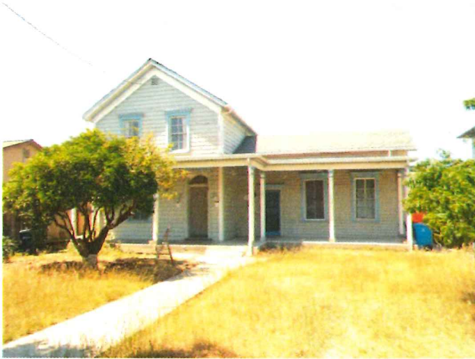
Photograph from 2014 showing differed maintenance
