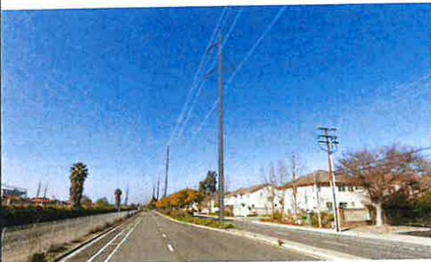
Facing North near Eisenhower Drive
