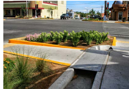
5.2.2.2 - Directional Ramps with ADA Access
