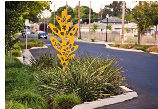
5.2.3.8C - Stormwater Planters in Parking Bulbout
