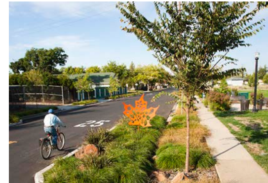
5.2.3.8B - Stormwater Planters in Bulbout
