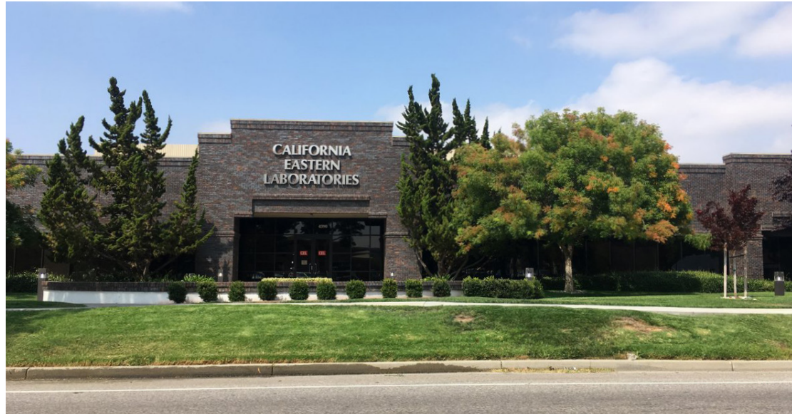
A Single-story Building Set Back from the Street
