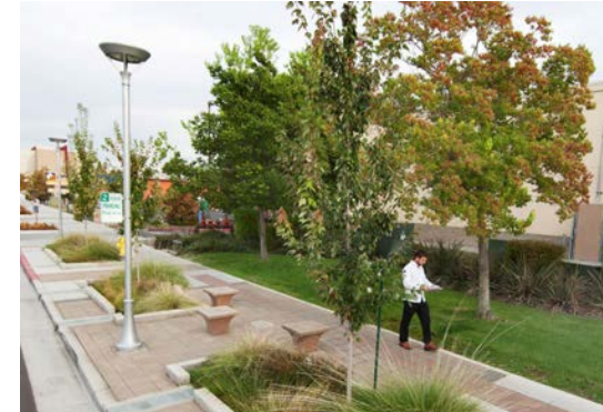
5.2.3.8A - Stormwater Planters in Pedestrian Zone
