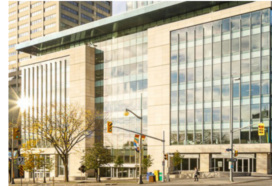
5.6.2.15A - Building Articulation to Break Up Façade
