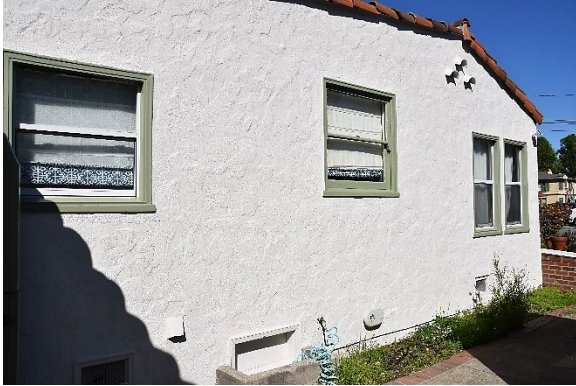
Figure 6. South façade, view northeast
