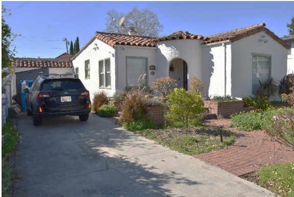
Figure 4. East façade, view northwest
