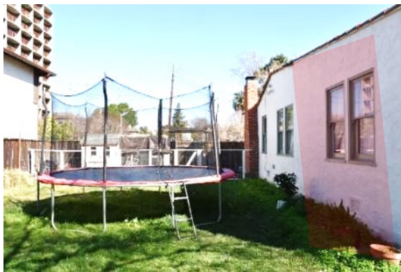
Figure 15. Views showing approximate location of materials/features to be removed (shaded pink) to accommodate the new addition.
