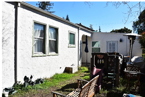
Figure 10. West façade of house (left) and north façade of garage (right), view southeast.
