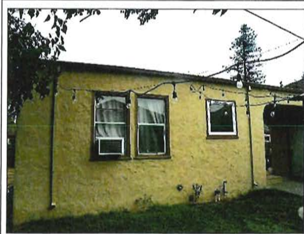
Photo No: 100_2701; View: Rear Façade. Photo Date: Sept., 2020; Camera Facing: E.
