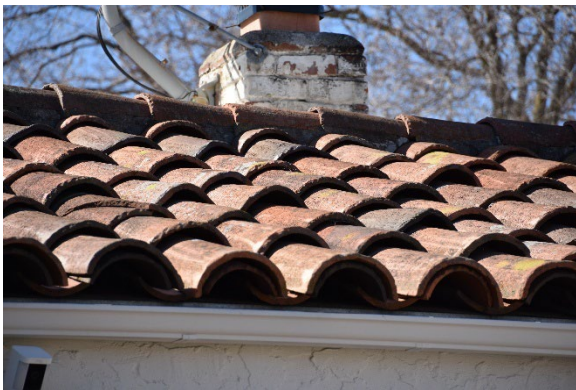
Figure 13. Detail of red roof barrel tiles.
