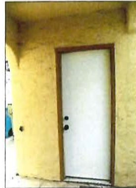
Photo No: 100_2716; View: Garage Man-door; Photo Date: Sept., 2020; Camera Facing: SE.
