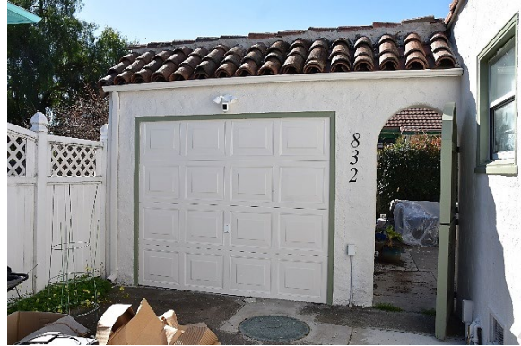
Figure 7. East façade, south end (garage) and arcaded wing wall detail
