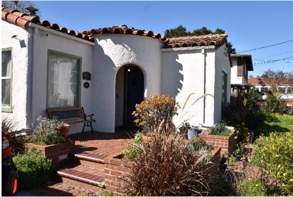
Figure 11. East façade, view towards tower and prominent arch at entry.
