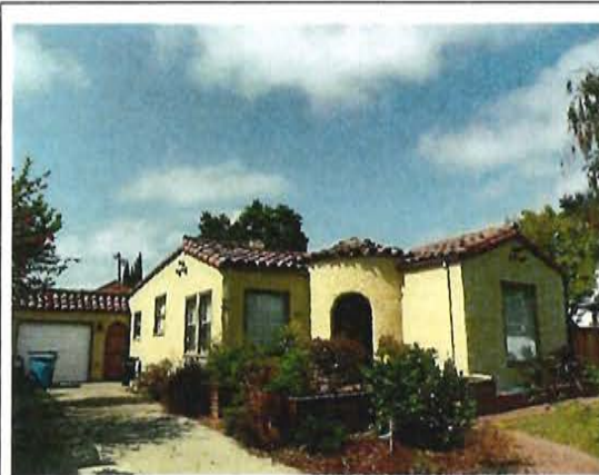
Photo No: 100_2732; View: South side-elevation and Front façade from Main street. Photo Date: Sept., 2020; Camera Facing: West.
