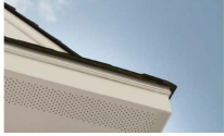
James Hardie Soffit Fiber Cement Vented Smooth Panel painted black satin finish 2X10 FASCIA JAMES HARDY - WITH ROYAL MOLDING
