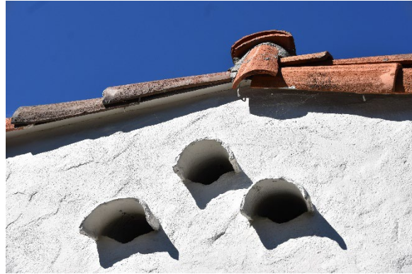
Figure 12. Detail of stucco wall, tile weep holes and red roof tiles.
