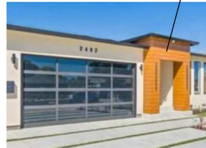
FRONT PORCH WOOD SIDING MATERIALS
