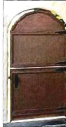
Top: Photo No: 100_2699; View: Arcaded Wing Wall door (arched solid wood plank with iron strap hinges); Photo Date: Sept., 2020; Camera Facing: WSW.
