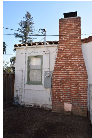
Figure 14. Detail of exterior brick chimney on north façade.
