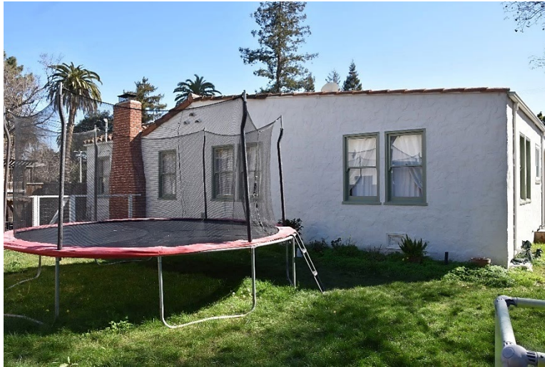
Figure 8. North façade, view southwest
