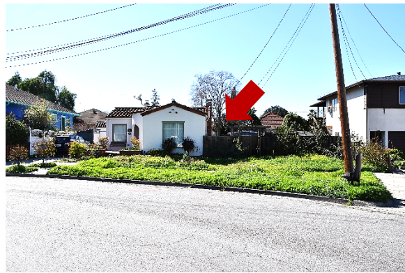
Figure 20. View west from Main Street.
