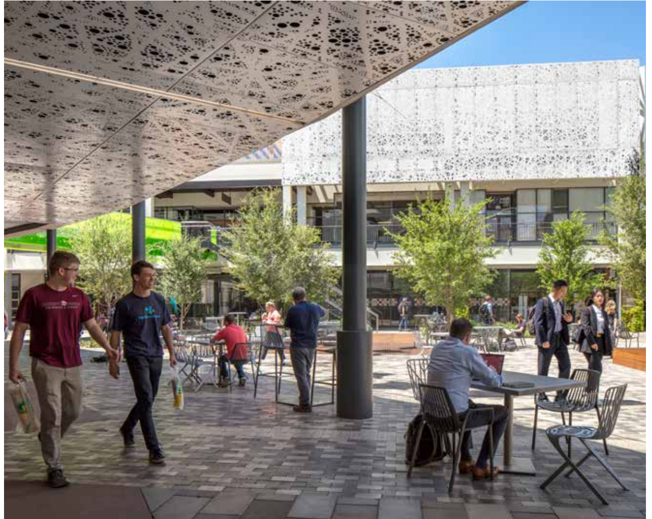
Arizona Center Refresh / Phoenix, AZ, US / Gensler
