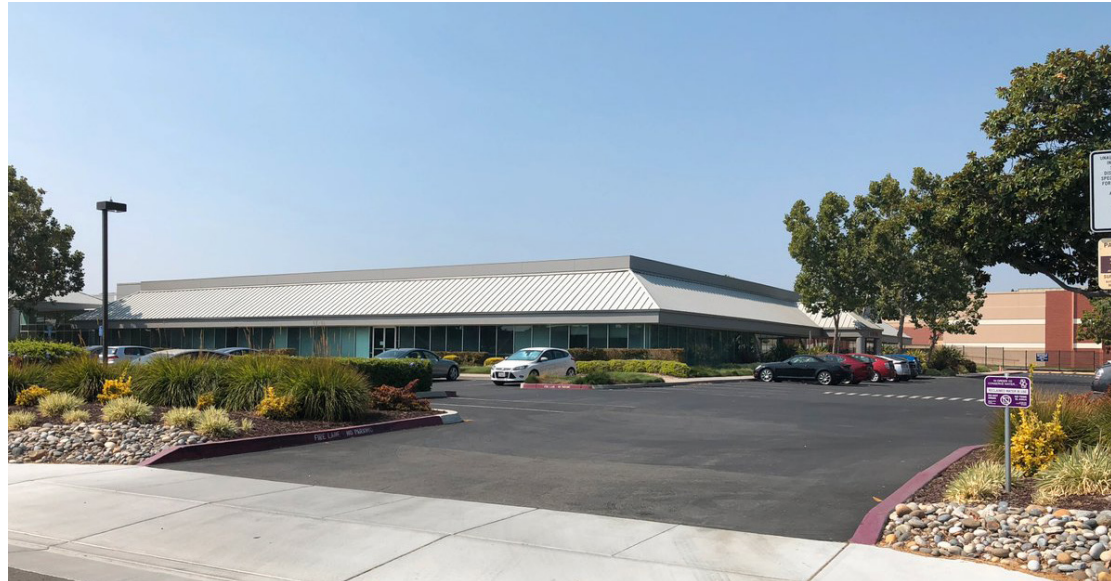
Low-density Office Building on Patrick Henry Drive
