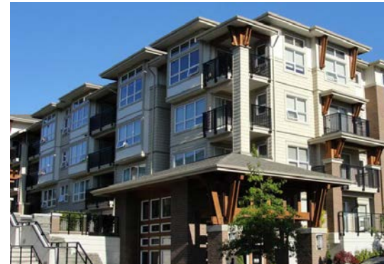
5.6.1.4 - Variation in Roof Lines
