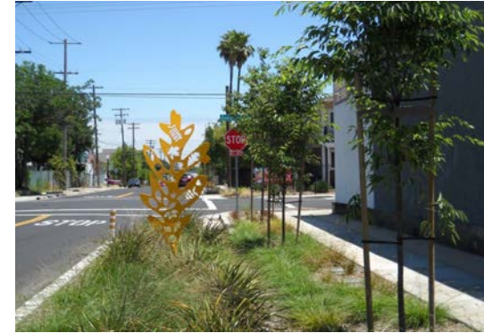
5.2.3.1 - Planters Along the Edge of Curb
