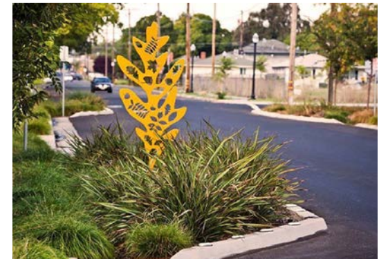
5.2.3.8C - Stormwater Planters in Parking Bulbout
