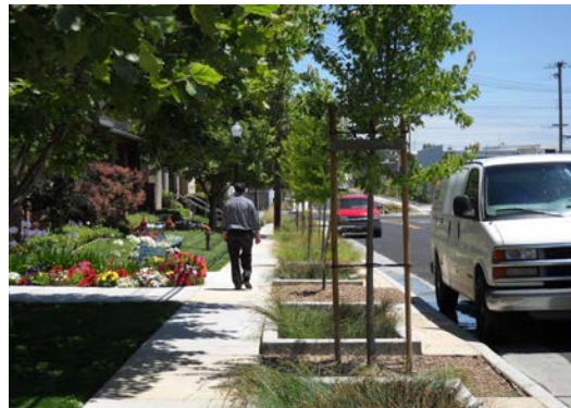
Planter Wells Between Sidewalk and Roadways
