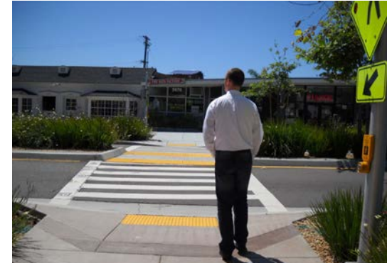
5.2.2.1 - Three-foot Deep Detectable Warning Surface
