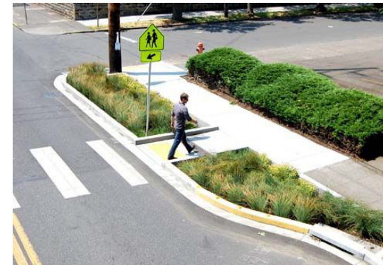
5.1.5.4 - Bulbouts at Intersection
