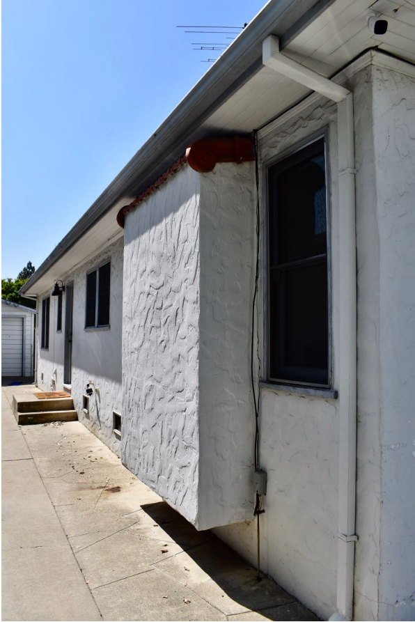
Three photos of the left side of the house. Top left: Looking toward the rear. Bottom left: Looking toward the front. Above: Terra cotta cap to the projection from the living room.
