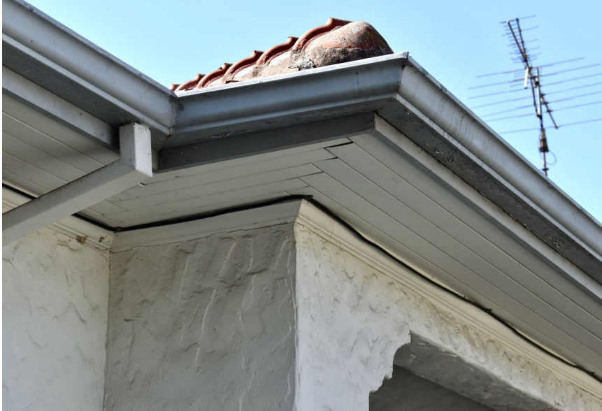
Above: Boxed roof eaves.
