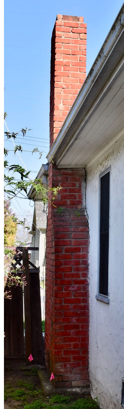
At right: Chimney on the right side of the house.
