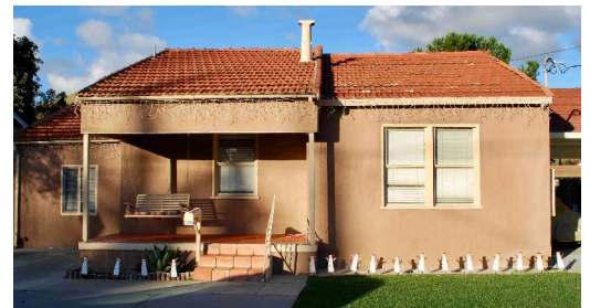
36708 Niles Boulevard (roof tiles since removed)
