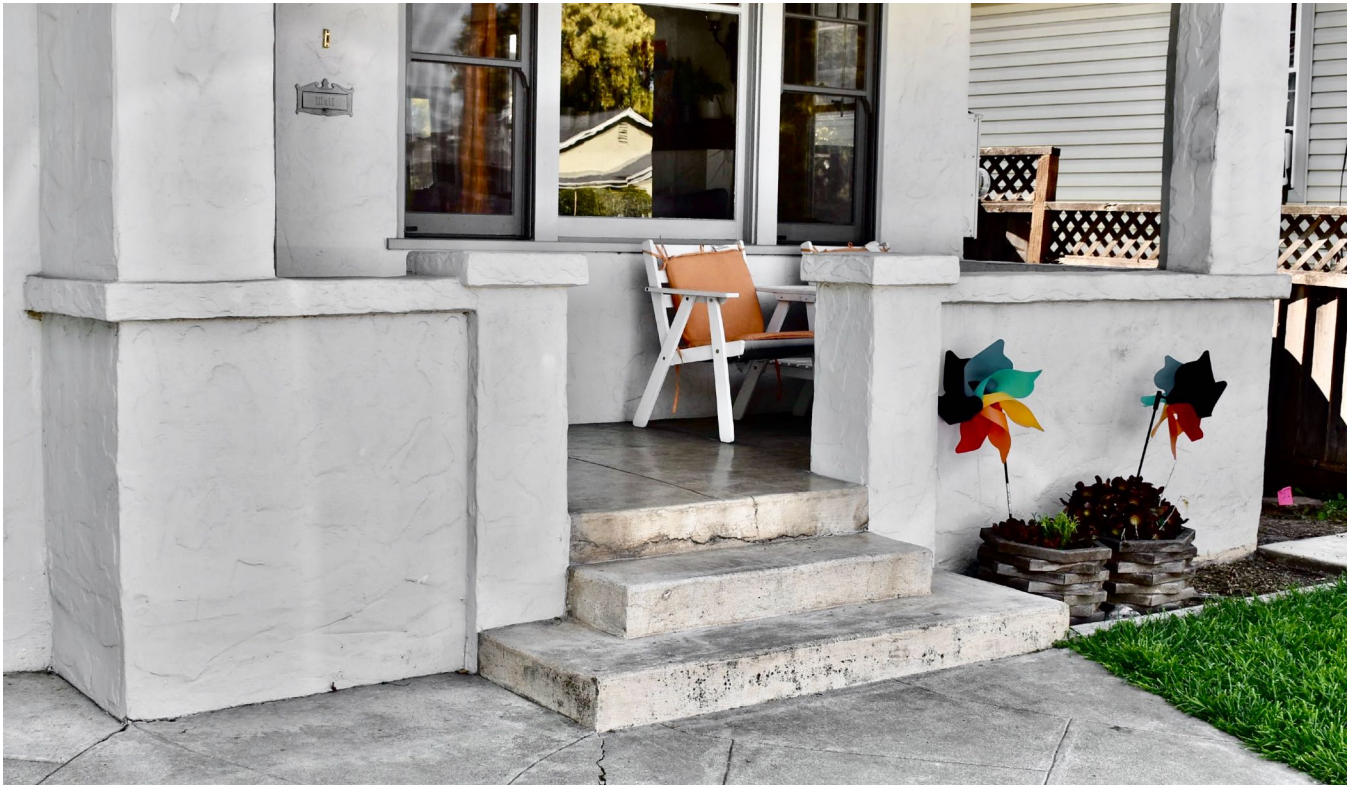
Above: The base of the porch. Its polished concrete deck and steps contrast with the rough texture of the stucco.
