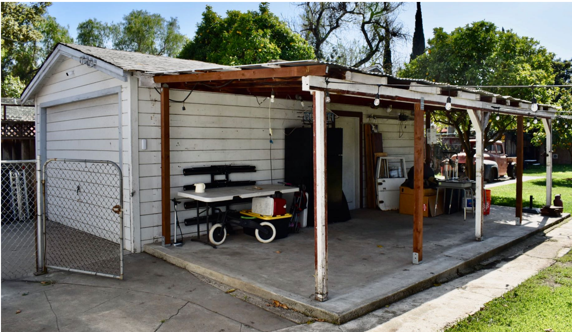
Below: The garage.
