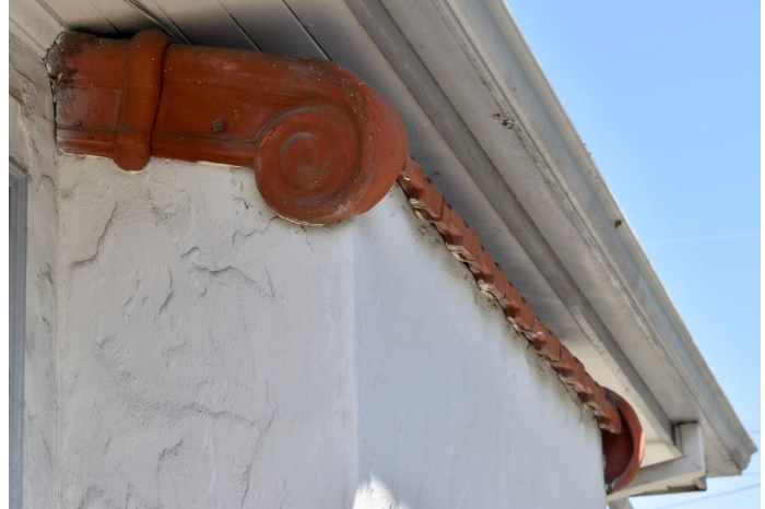
Three photos of the left side of the house. Top left: Looking toward the rear. Bottom left: Looking toward the front. Above: Terra cotta cap to the projection from the living room.
