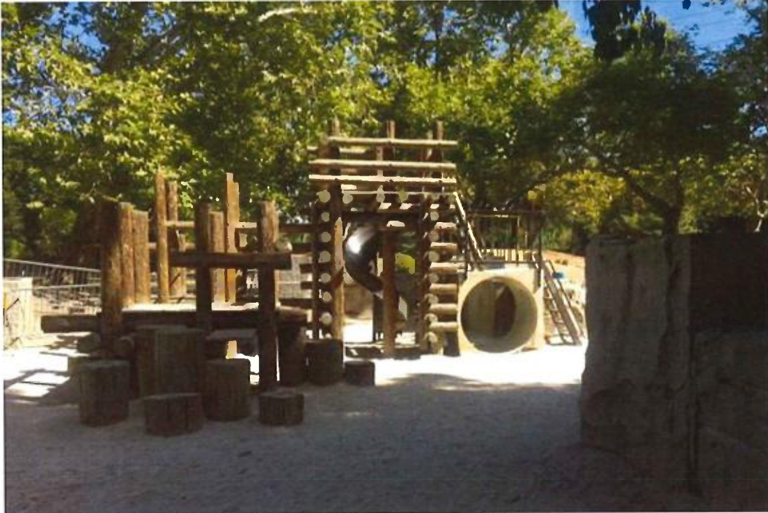
Existing Central Park Arbor Playground to be replaced. View facing east from Kiely Boulevard.
