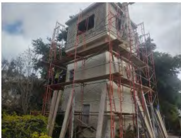
Repairs to Harris Lass
