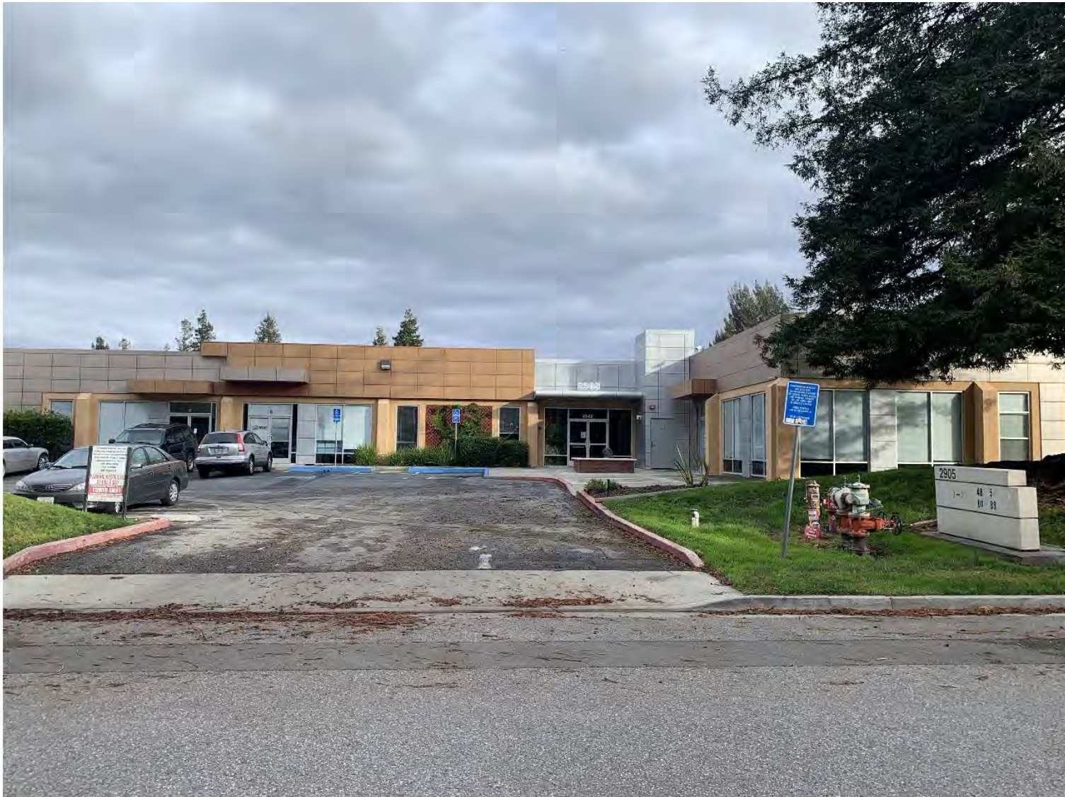
View of Project Site from West (Existing Conditions)
