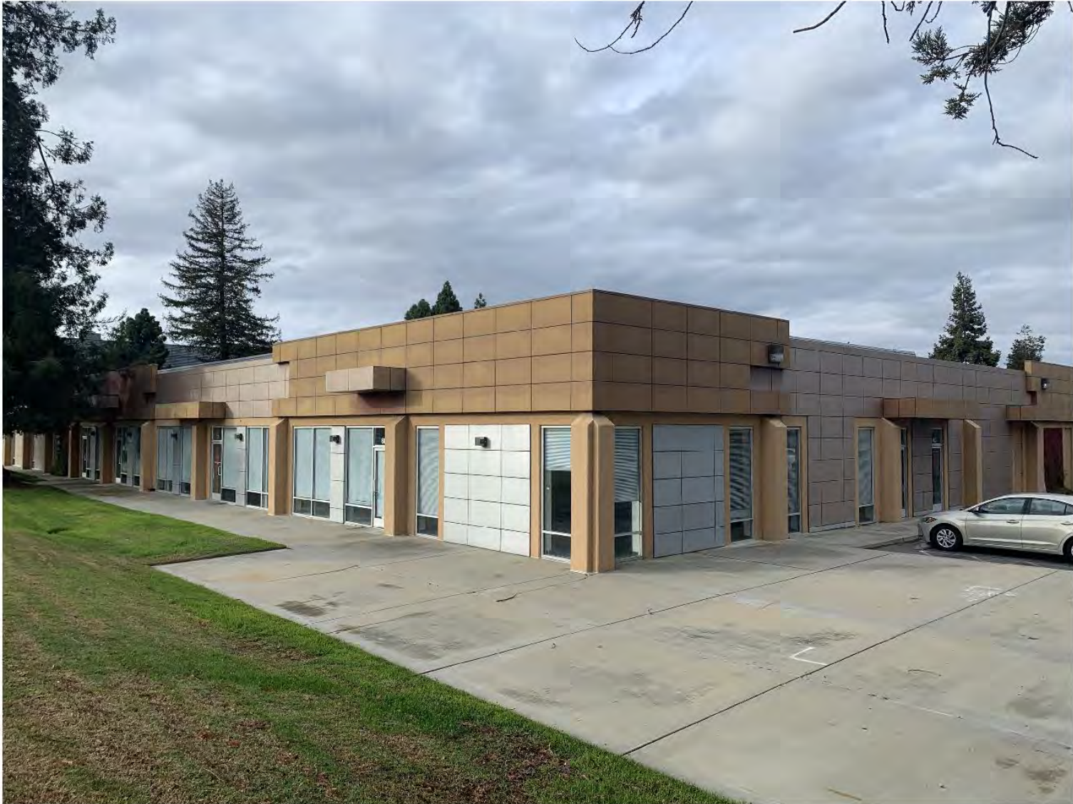
View of Project Site from Southeast (Existing Conditions)
