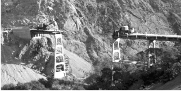
Construction at Anderson Reservoir, 1951
