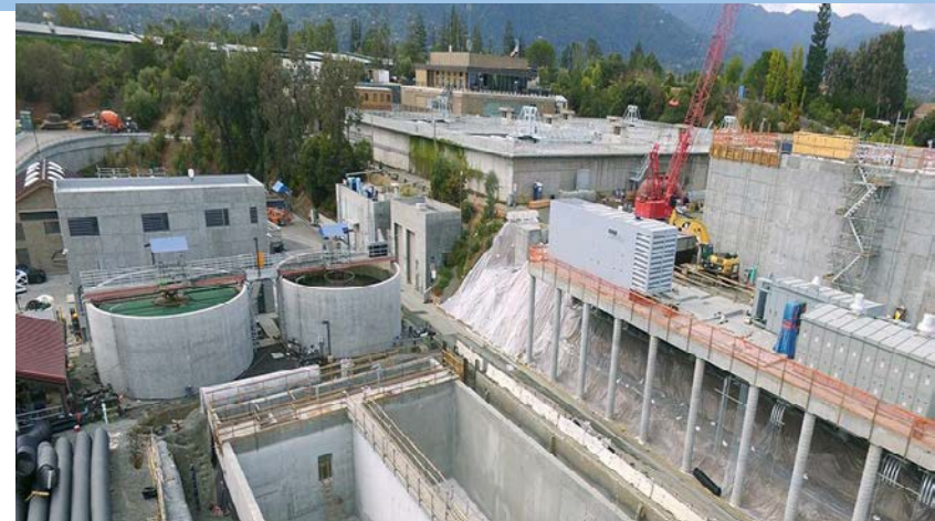
RWTP Reliability Improvements ($290 Million)
