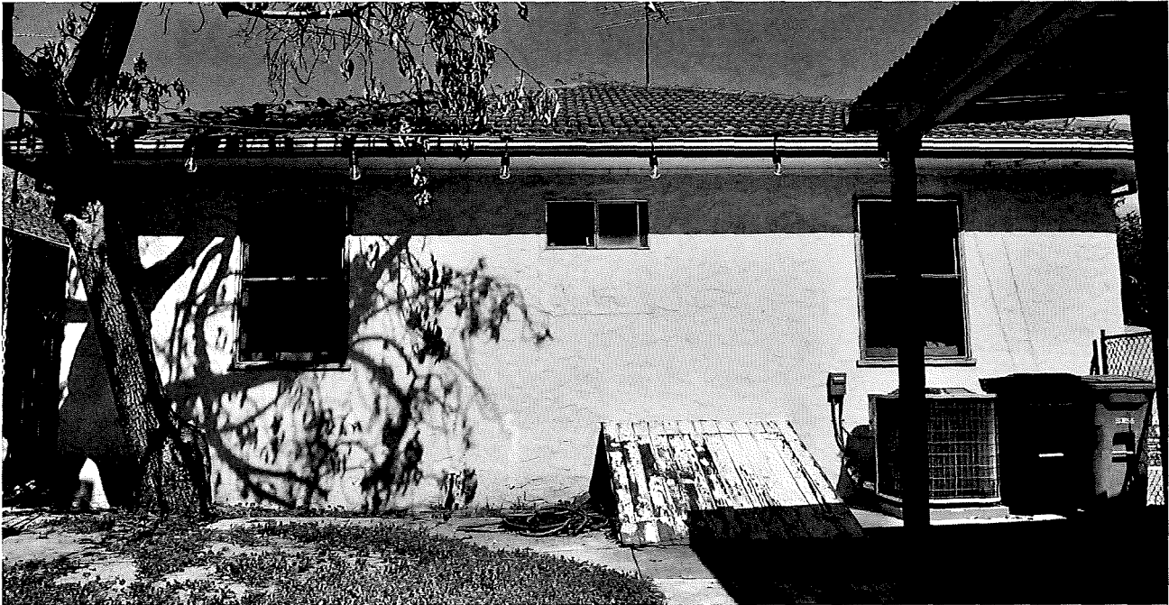
Above: The rear wall and roof of the house.
