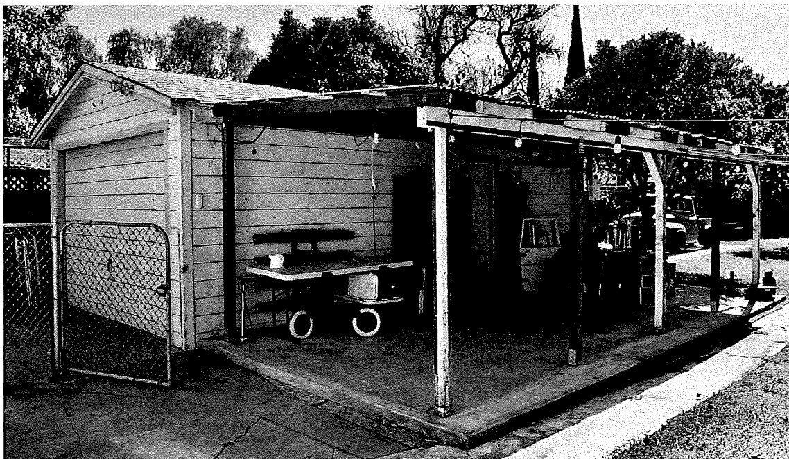
Below: The garage.
