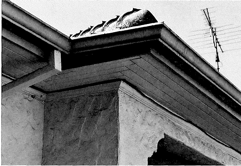
Above: Boxed roof eaves.
