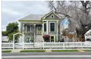
EXISTING PHOTO #P1
