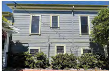
EXISTING PHOTO #P4
