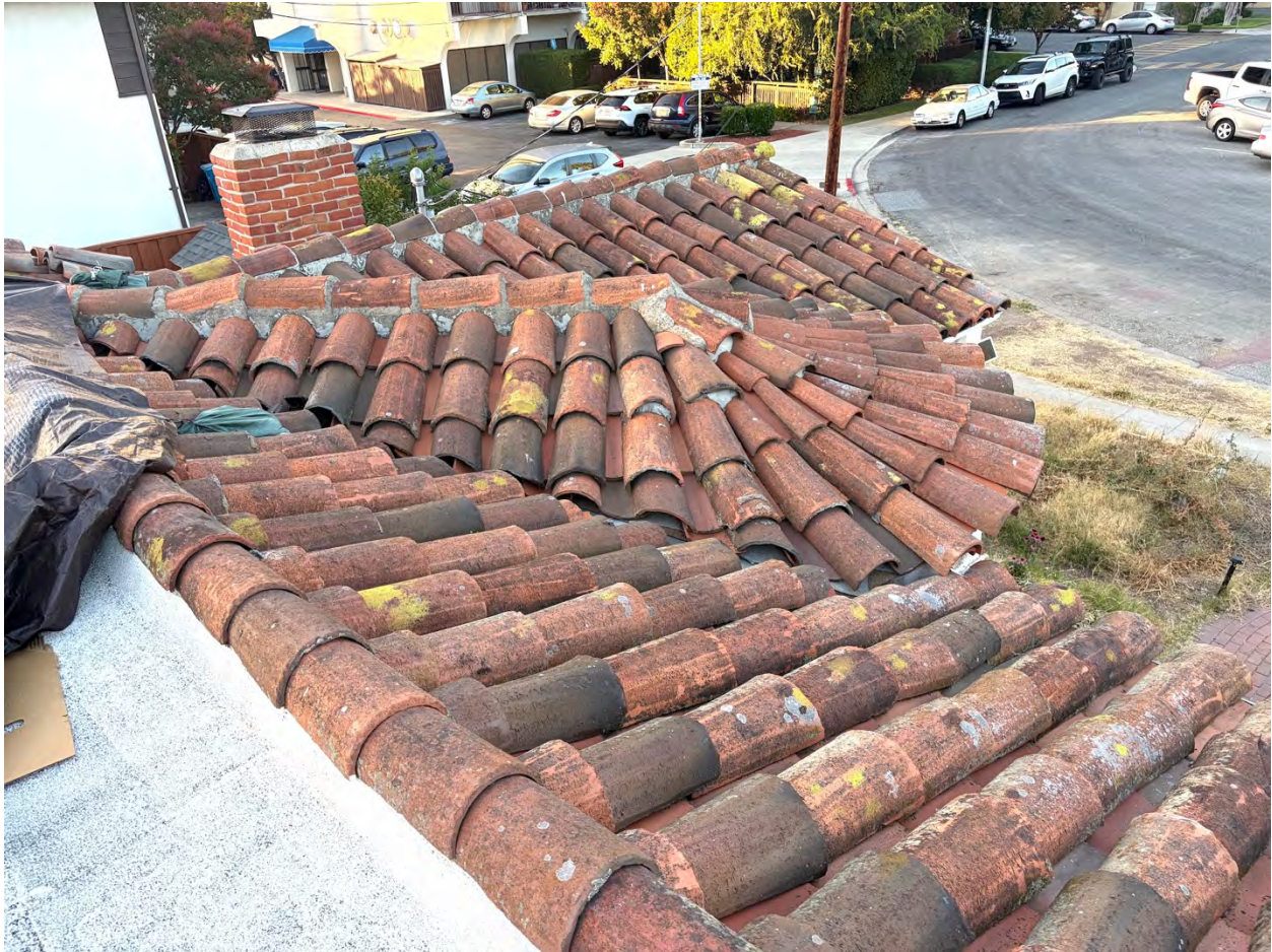
Figure 4. Roofing at main building of 834 Main Street (Andrew Fung, July 2026)
