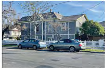
EXISTING PHOTO #P3
