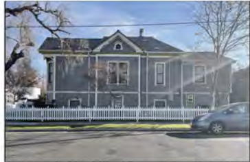
EXISTING PHOTO #P2
