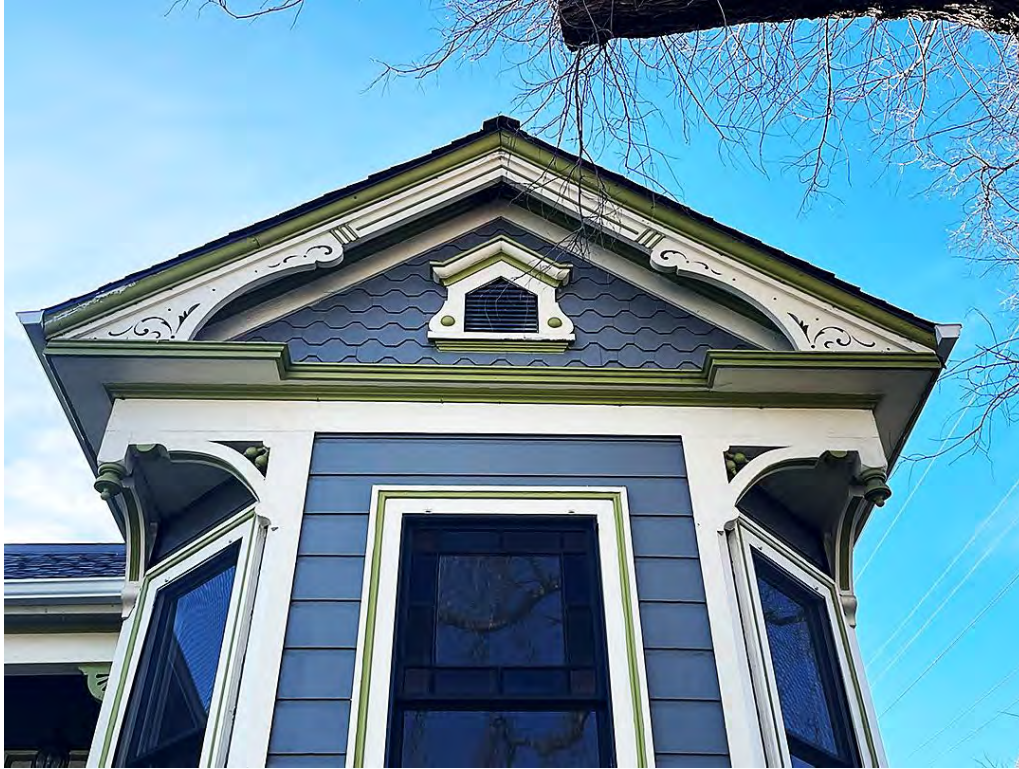
Figure 4: Victorian details in front gable.
