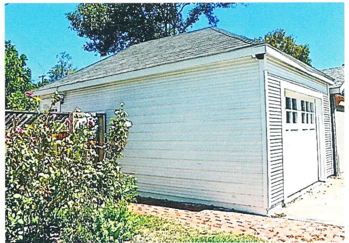
Photo No: 100_3059 View: Garage W side-elevation: August, 2022; Camera Facing: NE
