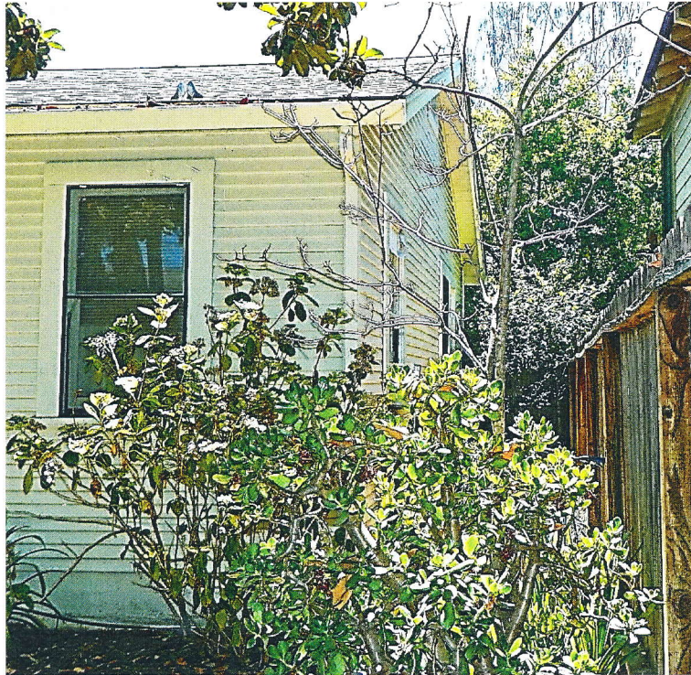
Photo No: 100-3083; View: Partial Rear Façade & W side-elevation; Photo Date: August 2022; Camera Facing: ESE
