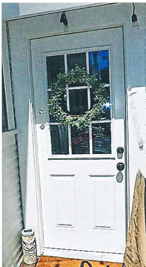
Photo No: 100_3063; View: Entry door into wing; Photo Date: August, 2022; Camera Facing: NNW
