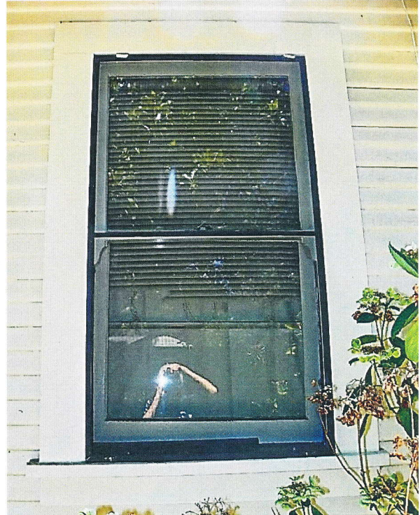
Photo No: 100_3089 View: Typical I-over-1 double hung window; August, 2022; Camera Facing: SSE
