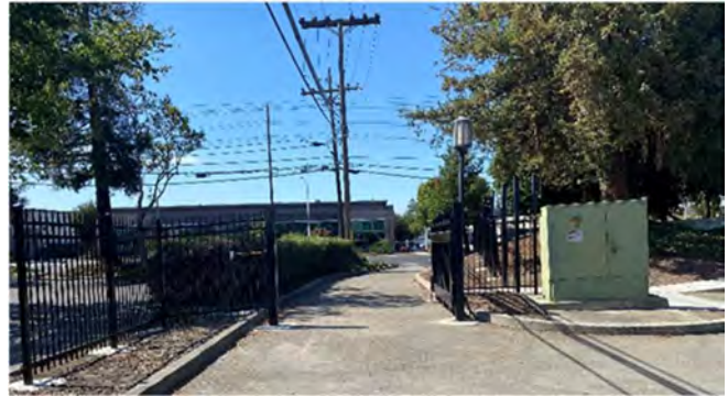
Emergency Operations Center Security Upgrades Project
