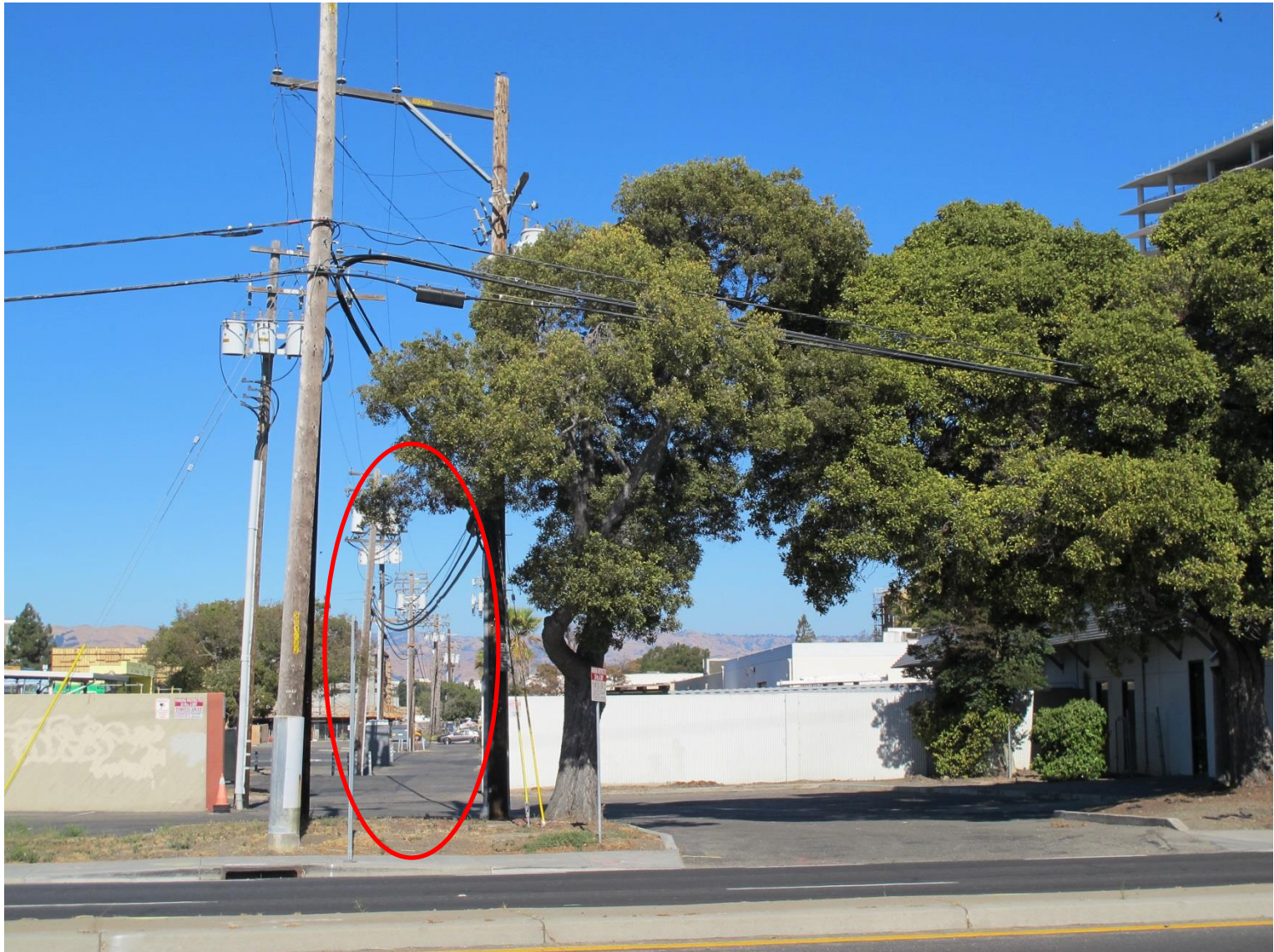
Figure 4: View from Lafayette down the alleyway between my building (on left) and proposed development (on right). Note power poles and droopy lines down the whole length of the alleyway (circled in red).
