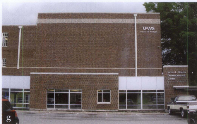
Figure 15. The rehabilitation of a c. 1930 high school auditorium for a clinic and offices proposed two additions: a one-story entrance and reception area on this elevation (a); and a four-story elevator and stair tower on another side (b). The gabled entrance (c) first proposed was not compatible with the flat-roofed auditorium and the design of the proposed stair tower (d) was also incompatible and overwhelmed the historic building. The designs were revised (e-f) resulting in new additions that meet the Standards (g-h).
