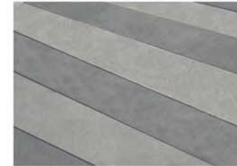
ENTRY PLAZA CONCRETE PAVING
