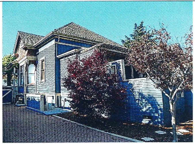
Photo No: 100_3404 View: S side-elevation from rear towards atreet Photo Date: December, 2023; Camera Facing: WSW.
