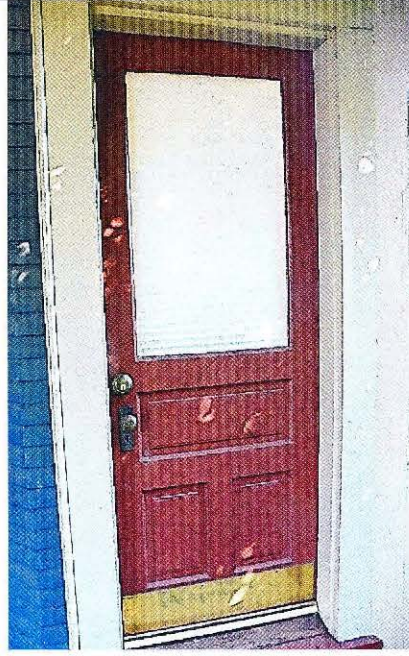
Photo No: 100_3358 View: Side Door Photo Date: 12/2023; Camera Facing: N
