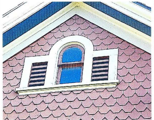
Photo No: 100_3353 View: Front gable Palladian window and louvered vents Photo Date: 12/2023; Camera Facing: ENE
