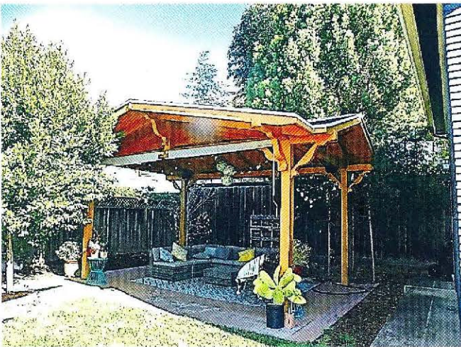
Photo No: 100_3413 View: Rear Yard Gazebo Photo Date: December, 2023; Camera Facing: NNE
