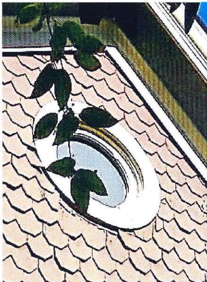
Photo No: 100_3396 View: Side gable window; Photo Date: 12/2023; Camera Facing: ENE
