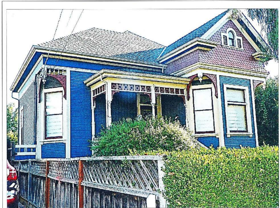
Photo No: 100_3308; View: Partial Front Façade & N side-elevation showing angled wall between Front and N side-elevation walls, with window, brackets, pendant and spindlework frieze; Photo Date: December, 2023; Camera Facing: ENE.
