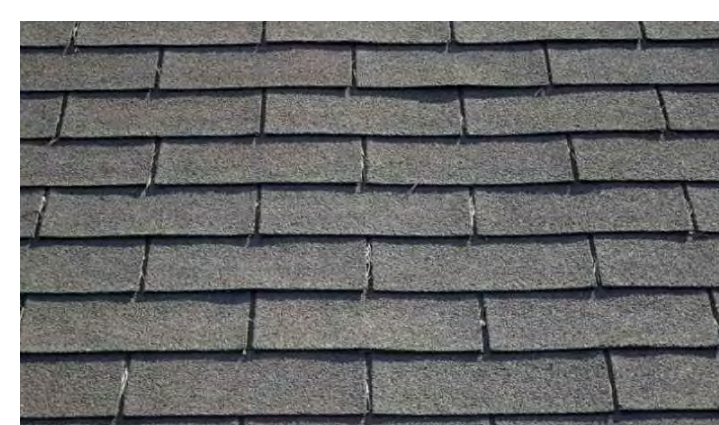
ASPHALT SHINGLE ROOF
