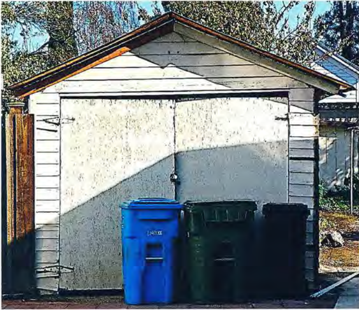
Photo No: 100_2901 View: Garage Front; Photo Date: December, 2021 Camera Facing: ENE
