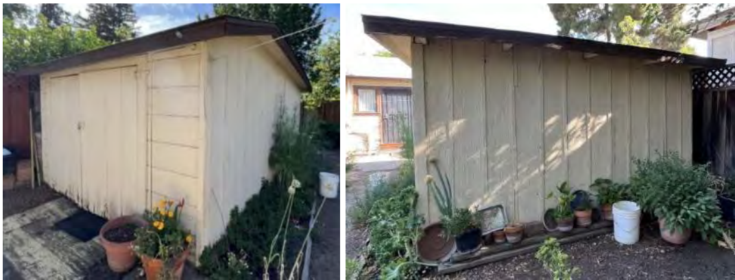
Figure 16. the garage to the south of the 1070 Lewis Street house.
