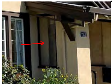
Phase: Design Comments: Window on porch is not original and should be removed.
