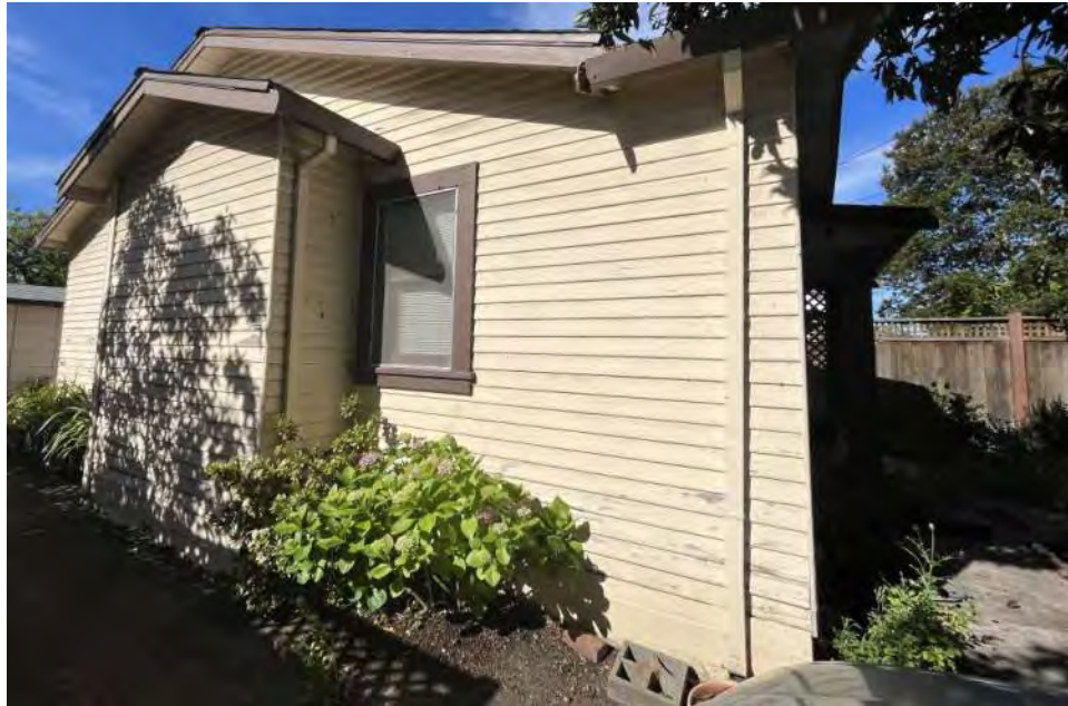
Figure 9. The east elevation of 1070 Lewis Street.
