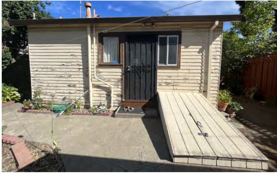
Figure 12. The south elevation of 1070 Lewis Street.
