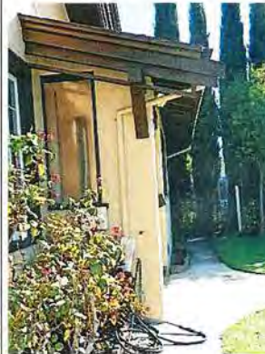
Left – Photo No: 100_2917 View: Front Porch roof trim; Photo Date: December, 2021 Camera Facing: SSE
