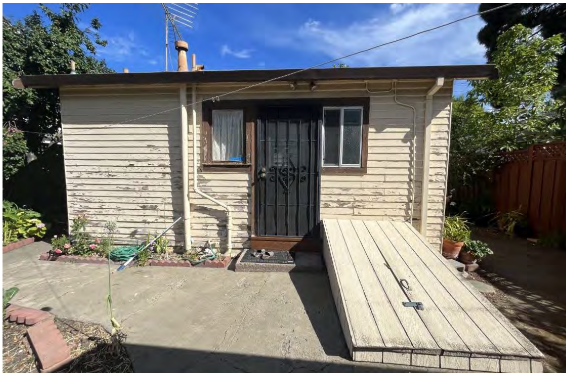
Figure 6. The south façade.
