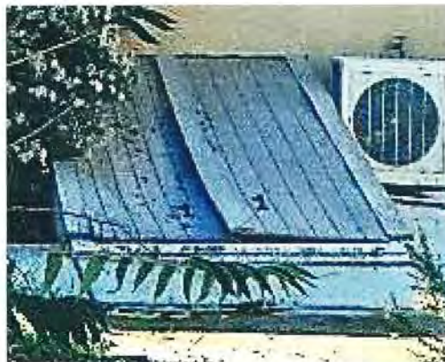
Photo No: 100_2005 View: Basement entry; Photo Date: December, 2021 Camera Facing: WSW
