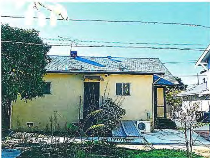
Photo No: 100_2905 View: Rear façade; Photo Date: November 2021; Camera Facing: WSW
