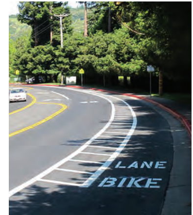
EXAMPLE OF BUFFERED BIKE LANES A buffer between vehicle traffic provides additional comfort for cyclists.
