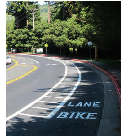
BUFFERED BIKE LANES A buffer between vehicle traffic provides additional horizontal separation from vehicles.
