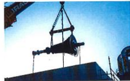
Steam Turbine Rotor
