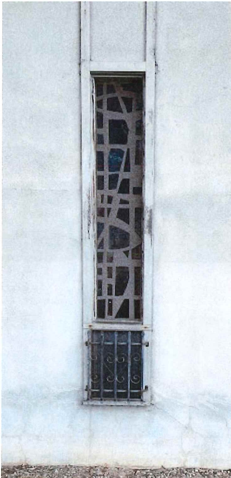
Photograph 10 1957 Pruneridge Avenue, Santa Clara View: window detail. On the left is a Blenko-style vertical window in a concrete setting. On the right is a section of the side window with wood mullions and wood frames.
