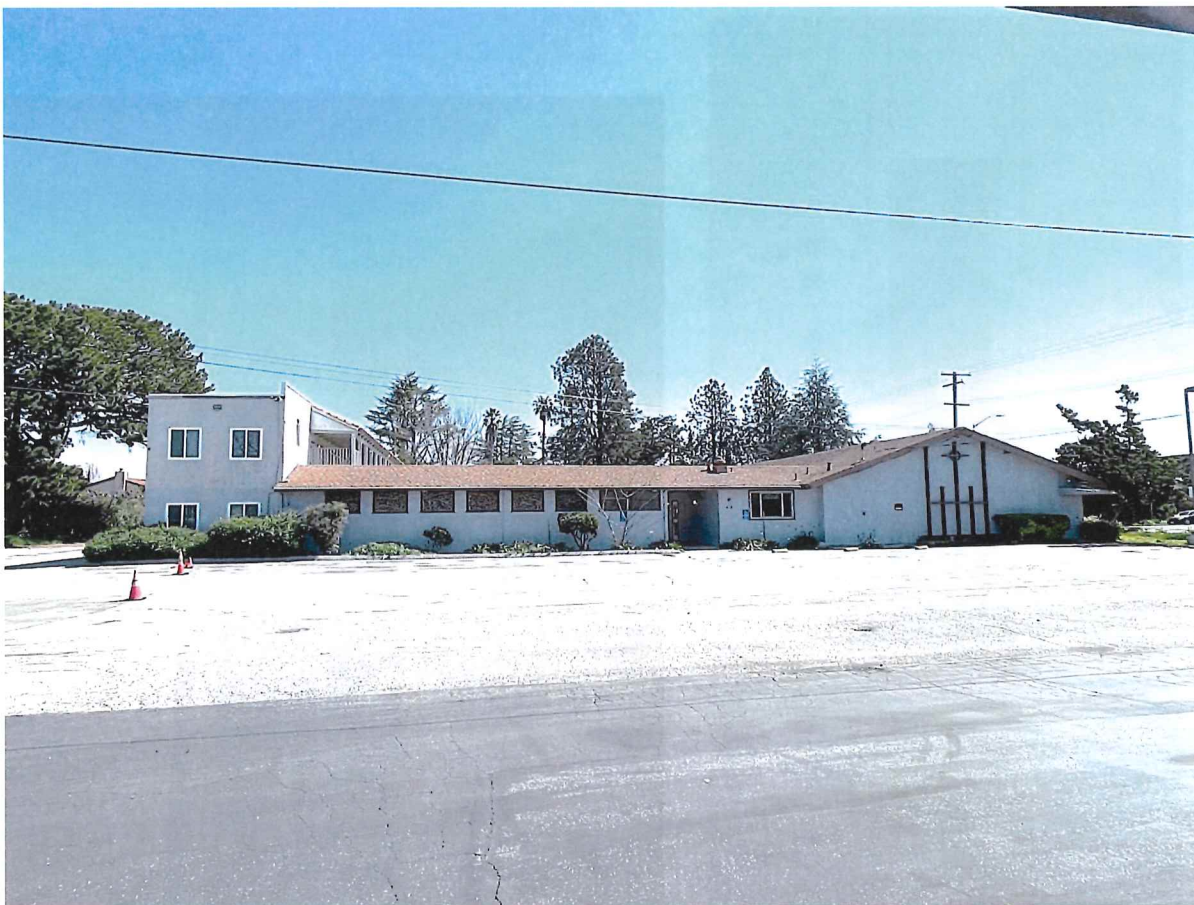
Photograph 11 1957 Pruneridge Avenue, Santa Clara View: Looking east at the rear of the classroom and parish hall complex.
