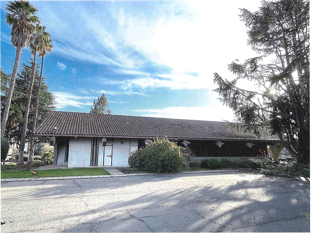
Photograph 4 1957 Pruneridge Avenue, Santa Clara View: North façade showing rear portion of the building with smooth stucco and vertical windows.
