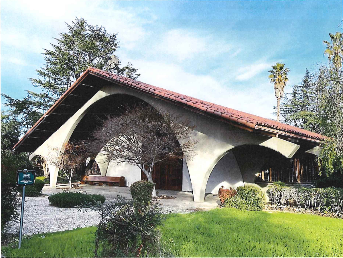
Photograph 2 1957 Pruneridge Avenue, Santa Clara View: Front façade showing the aggregate front patio and pad with the Concrete arch forming the covered entrance. Red tile curves over the eaves along the gable.
