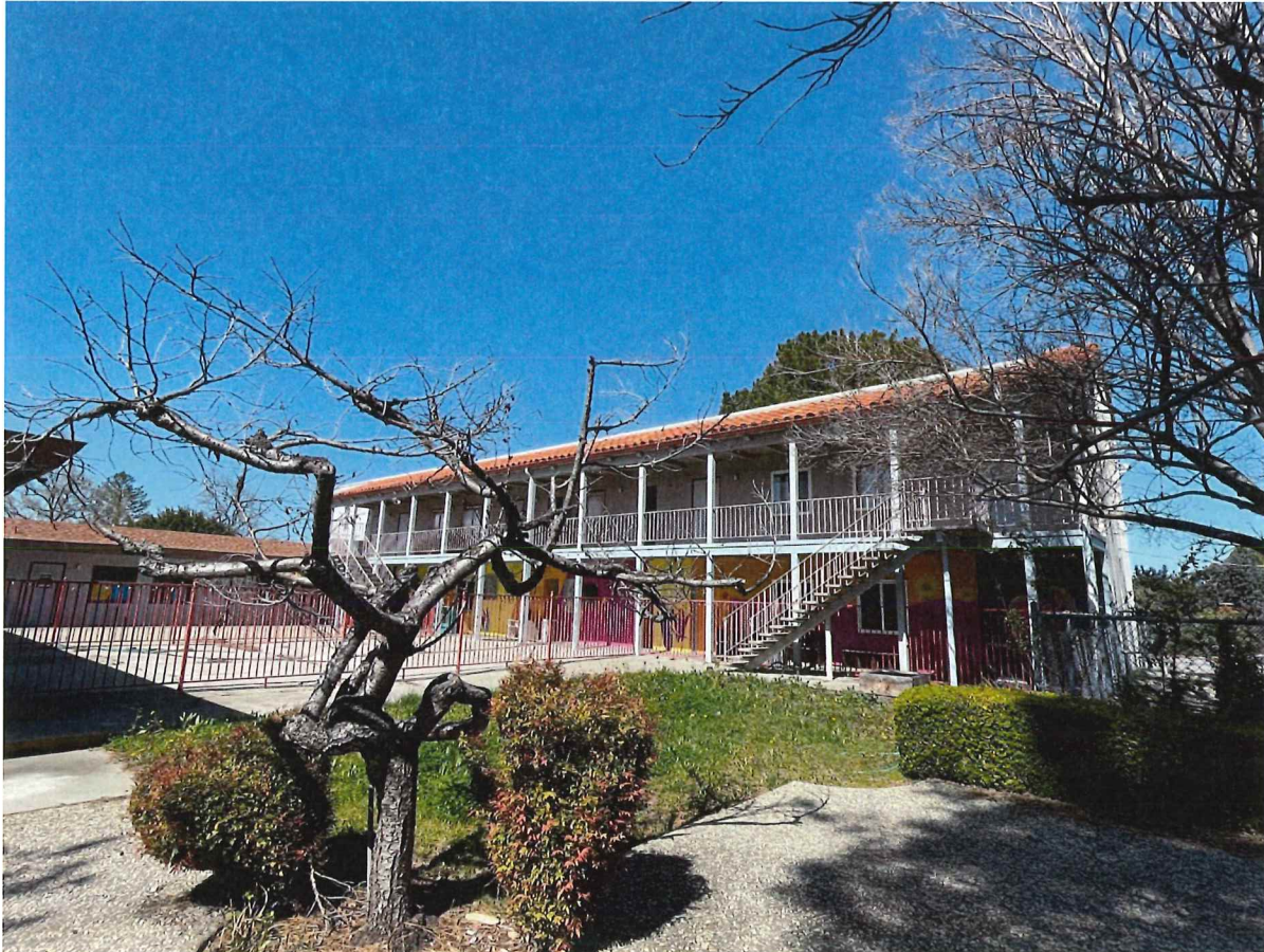
Photograph 14 1957 Pruneridge Avenue, Santa Clara View: The two-story classroom building that faces south in the courtyard.
