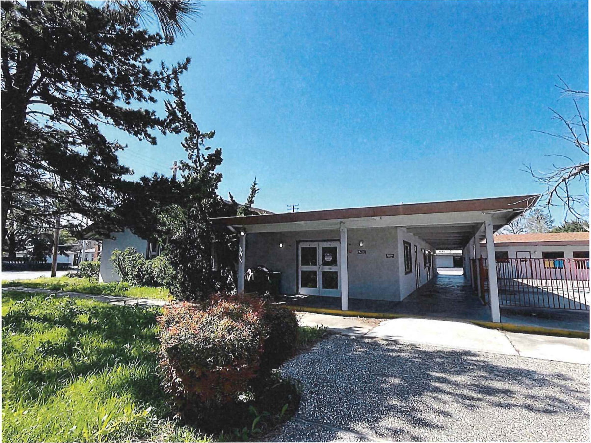
Photograph 13 1957 Pruneridge Avenue, Santa Clara View: Courtyard next to the Parish hall with a broad overhanging roof covering the walkway.
