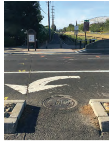
A C-15 MH 54-7 GROUND SURFACE
