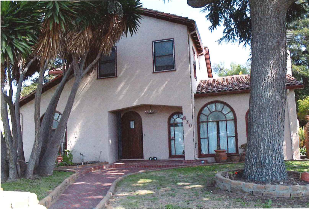
Photograph 2 820 Civic Center Drive
