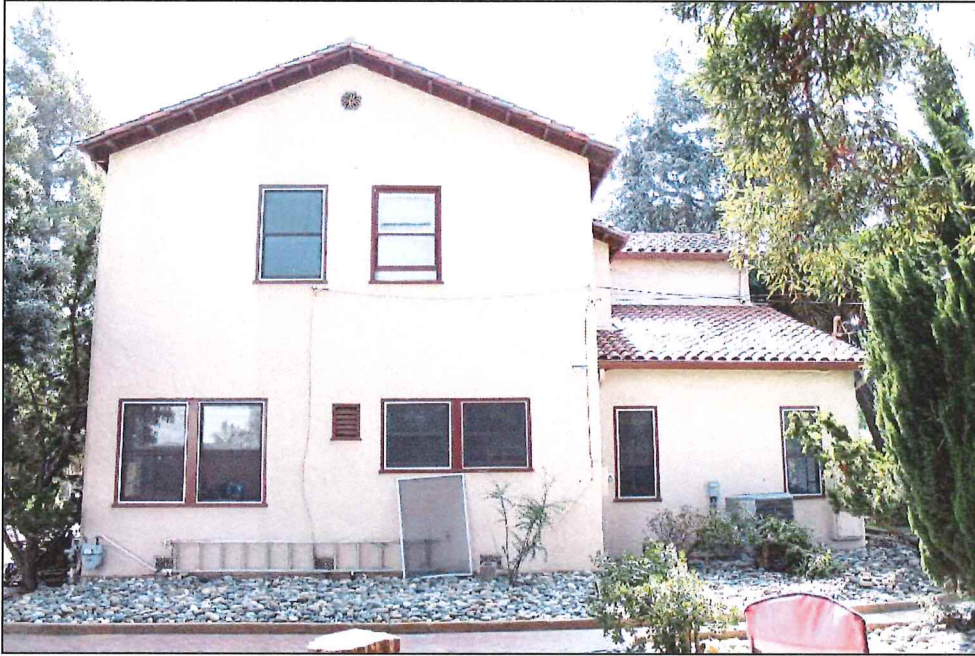
Photograph 3 820 Civic Center Drive
