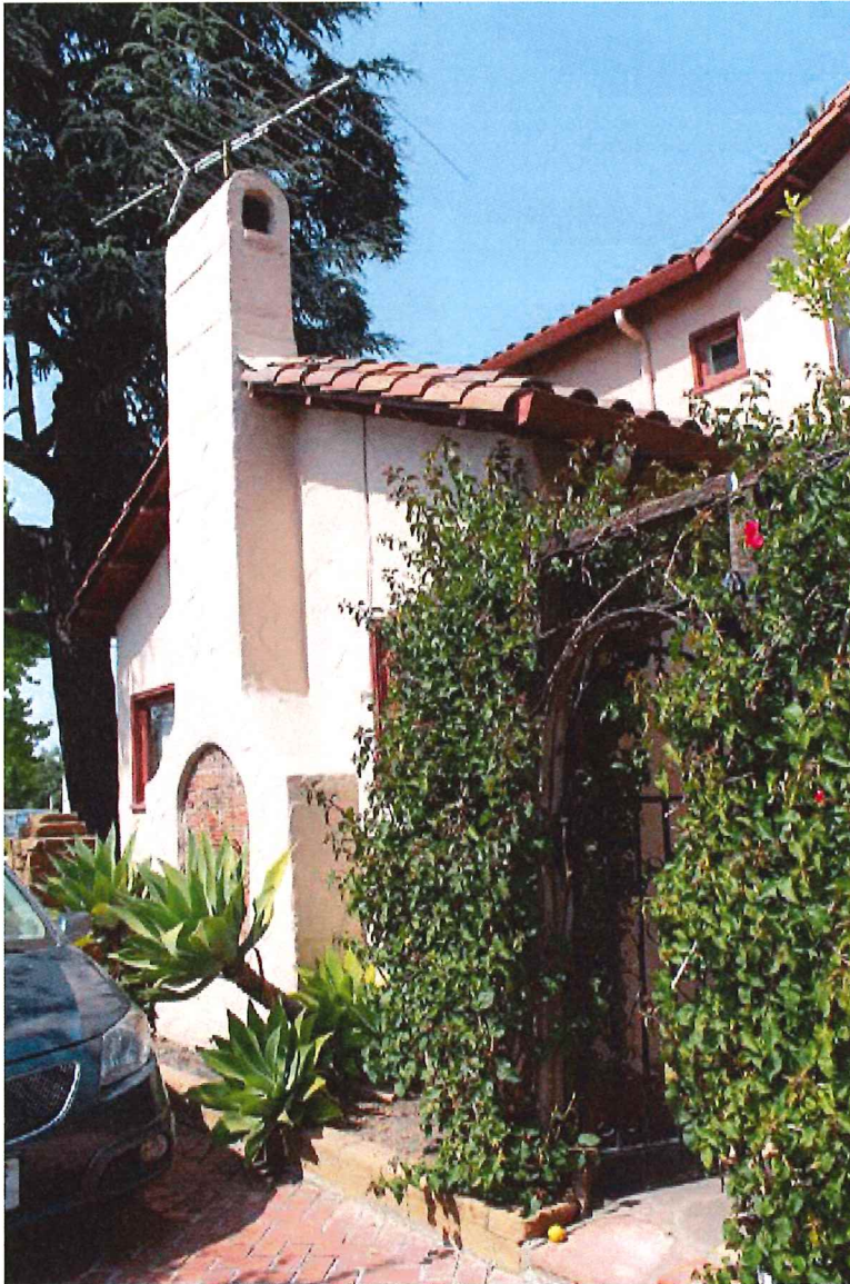
Photograph 6 820 Civic Center Drive View: West side façade, note articulation of the front sections, Chimney with brick inset at the base. Camera Facing: NE
