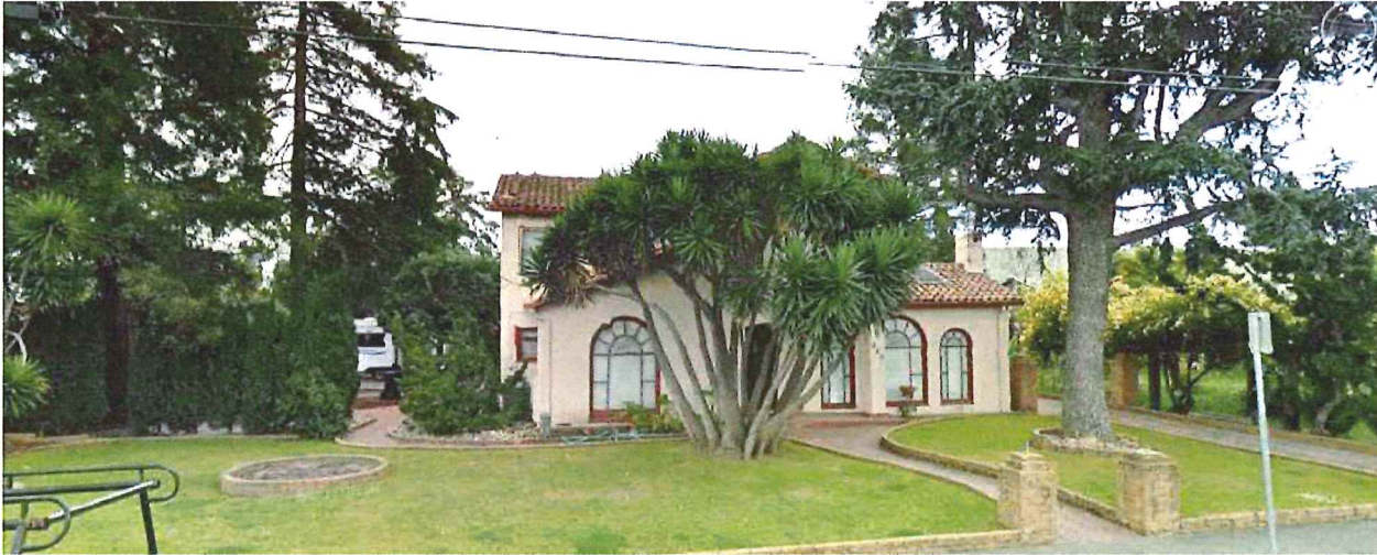
Photograph 1 820 Civic Center Drive.
