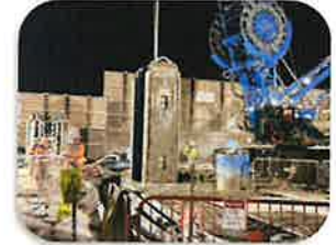
Excavation of "Tunnel Eye" – Wall Where Tunnel Boring Machine Will Start Boring
