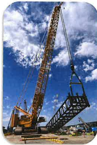
Test Lift of Rebar Cage Tripping Frame
