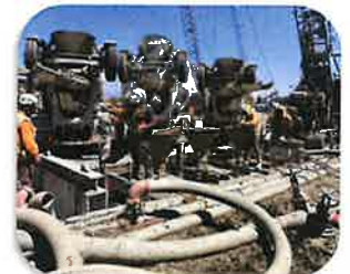
Concrete Placement for Support Walls
