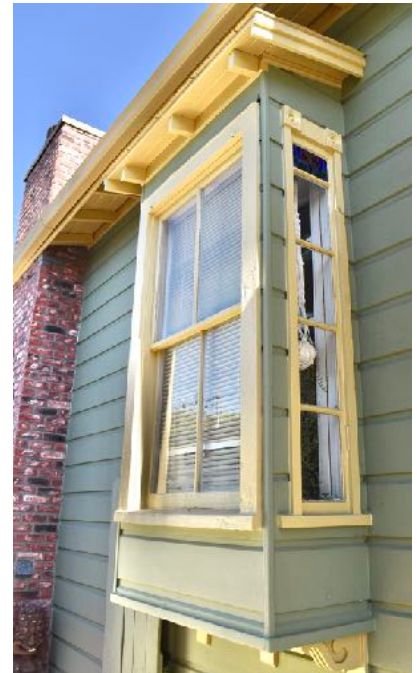
At left and below: Bay window with supporting brackets.
