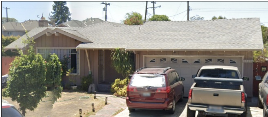
EXISTING ON SITE FRONT SITE VIEW A
