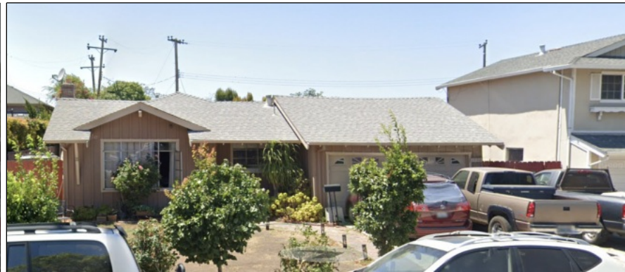
EXISTING ON SITE FRONT SITE VIEW B
