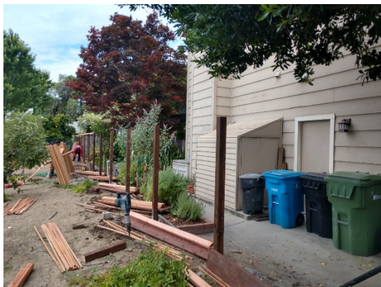
Morse Mansion Good Neighbor Fence Before
