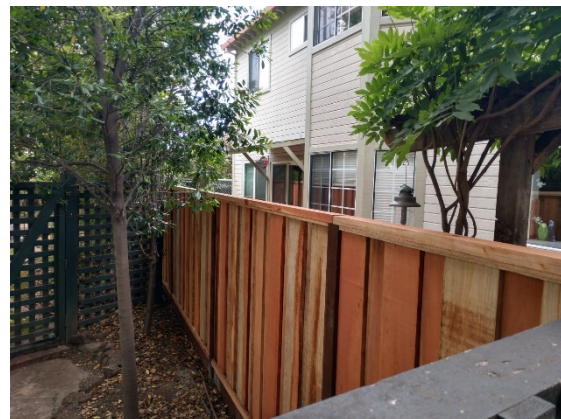
Morse Mansion Good Neighbor Fence After
