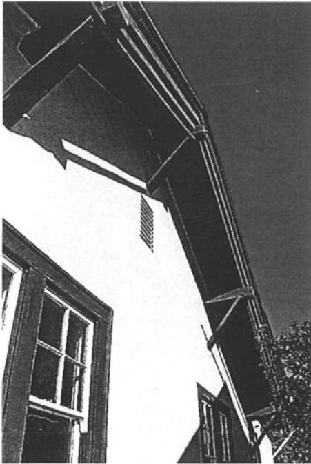
Photo No: 100_2916 View: S Side Gable, unenclosed eaves and knee braces; Photo Date: December, 2021; Camera Facing: NNE
