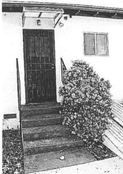
Photo No: 100_3005 View: Rear entry – (addition); Photo Date: December, 2021 Camera Facing: W
