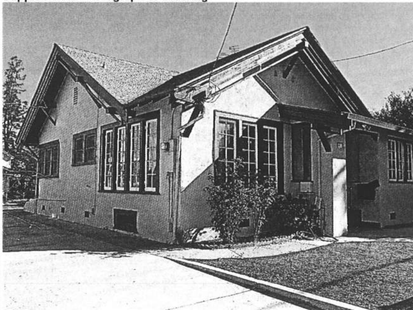
Description of Photo: (view, date, accession #) (Camera pointing E) North side-elevation and partial front façade. Photo No: 100_2894; 12/31/2021.
