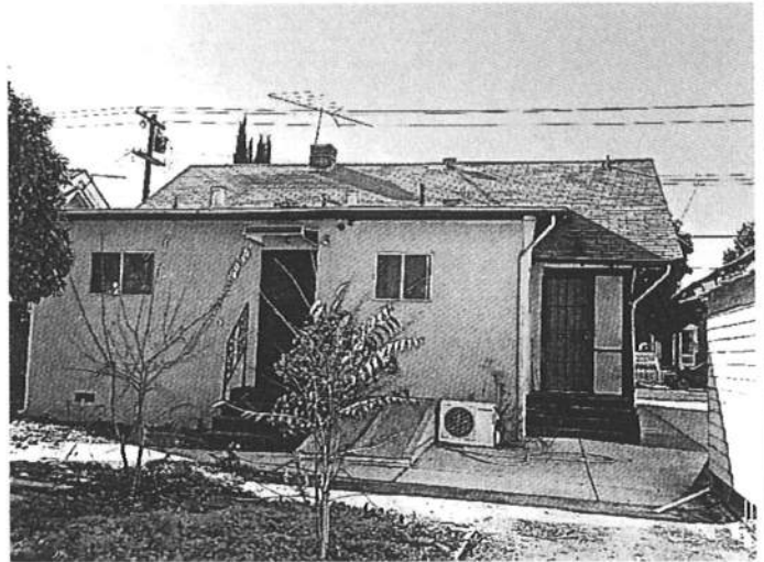
Photo No: 100_2909 View: Rear façade, view towards street; Photo Date: December 2021; Camera Facing: WSW
