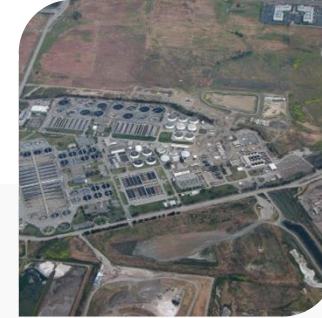
Regional Wastewater Facility
