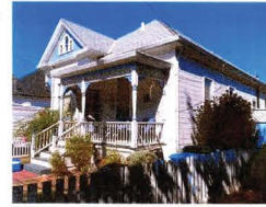
Photograph 2 1277 Jackson St. View: Front facade and right side wall. Note the raised level of the porch and first floor.
