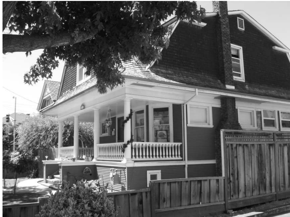
Photo 11: Oblique view of northeast corner of the residence.
