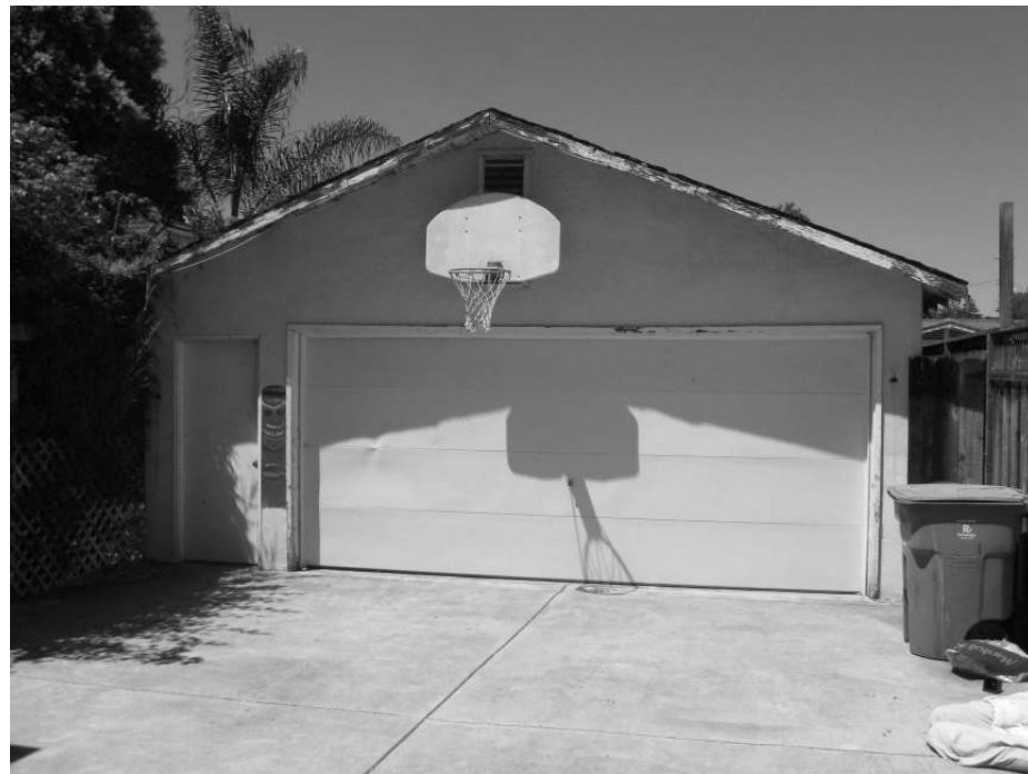
Photo 19: View of the detached garage, constructed 1971.
