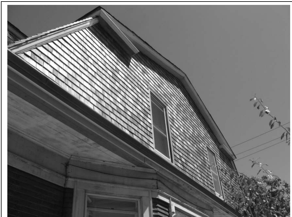
Photo 19: View of the cross-gambrel on the southern façade.
