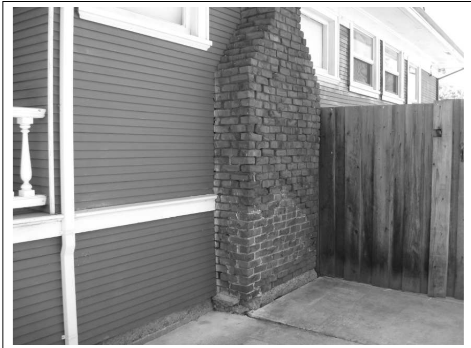
Photo 14: View of base of the chimney on the northern façade.
