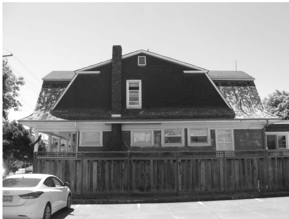
Photo 12: View of the northern façade from the adjacent lot.
