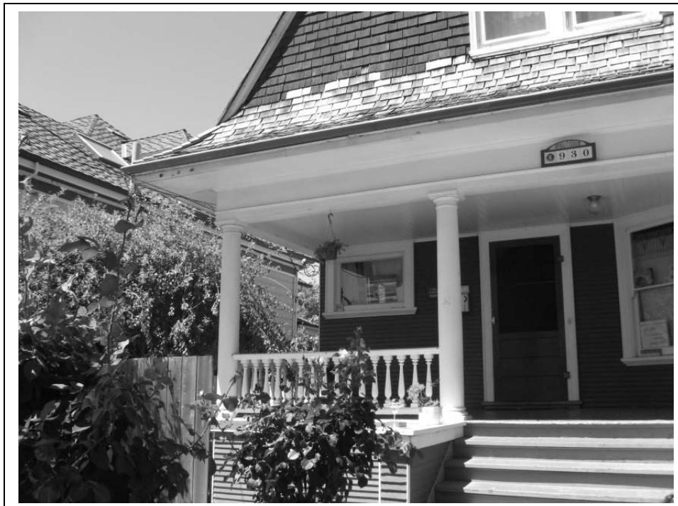
Photo 5: View of the southern side of the 1 st story front façade..
