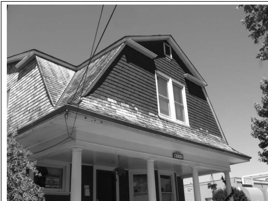
Photo 9: Oblique view of the front gambrel from the southeast.
