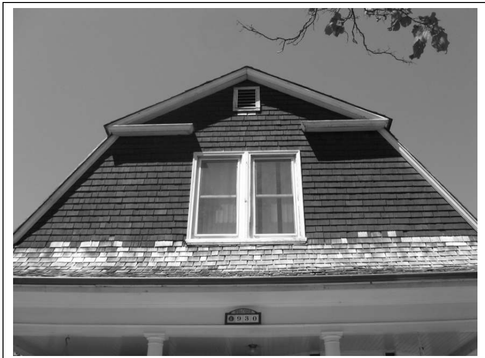
Photo 3: View of the front facing gambrel and dormer window.
