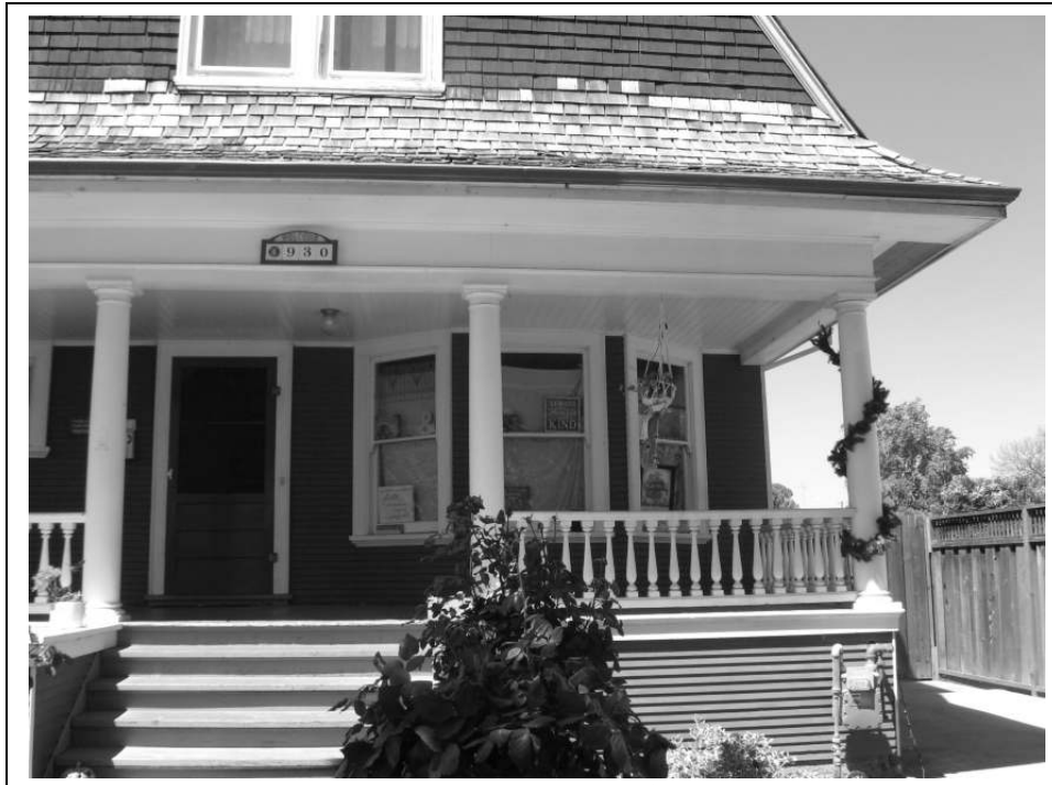
Photo 6: View of the northern side of the 1 st story front façade.
