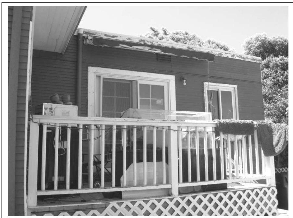
Photo 18: View of the rear addition from the north.
