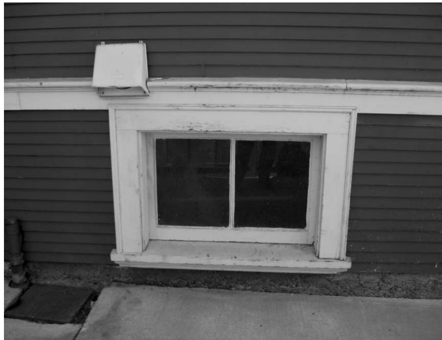
Photo 15: View of wooden framed basement window on north façade.
