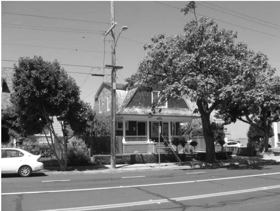
Photo 1: View of the front facade of the residence at 930 Monroe Street.
