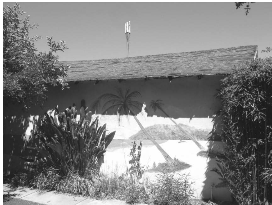
Photo 20: View of the southern façade of the garage showing mural.
