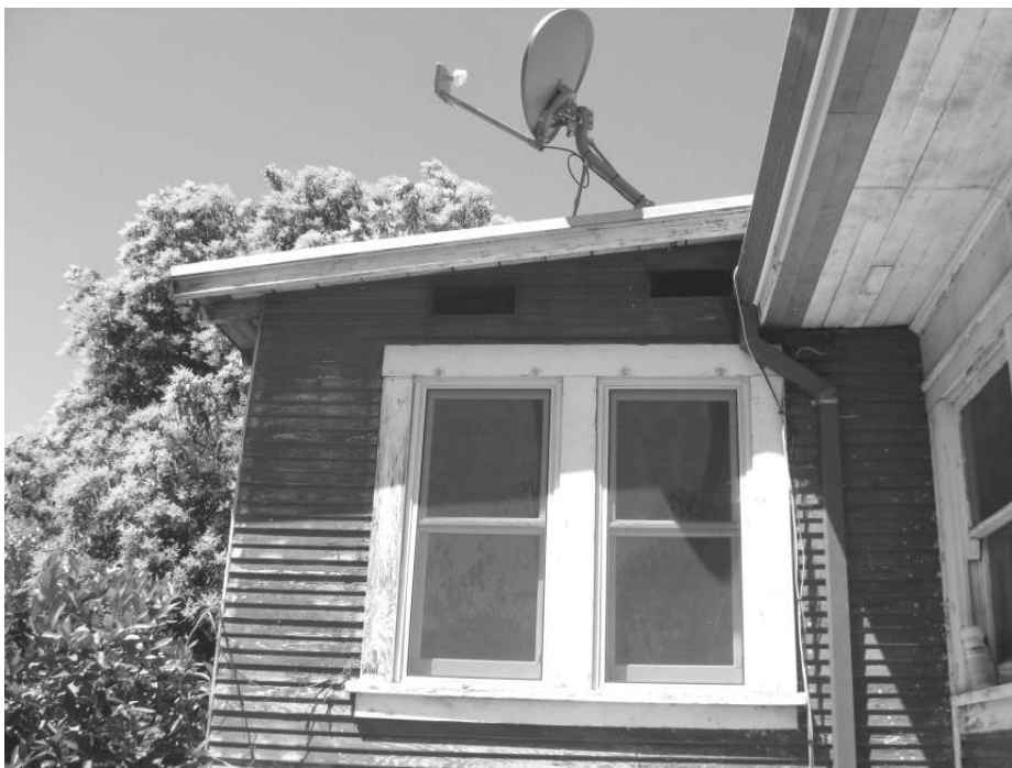
Photo 20: View of wooden framed windows on the rear addition.
