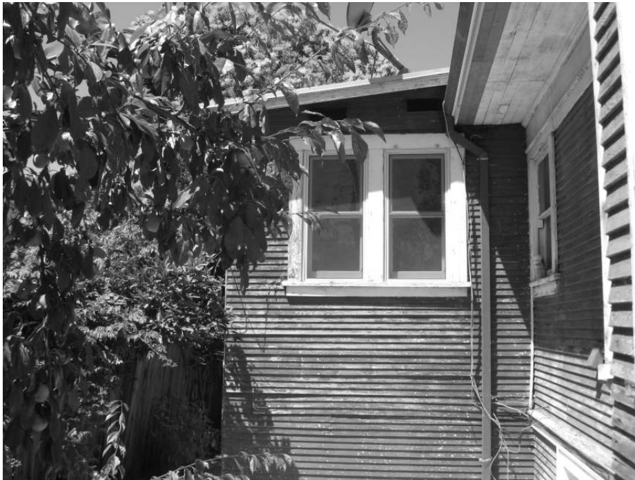
Photo 19: View of the southern portion of the rear addition.
