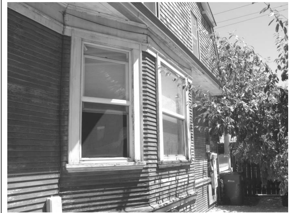
Photo 20: View of bay windows on the southern façade.
