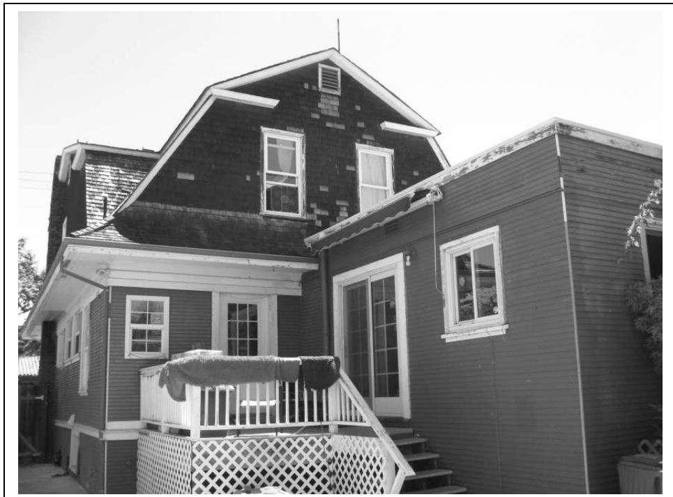
Photo 19: Oblique view of the residence from the northwest.
