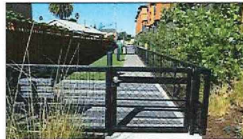
Pet Area & Entry Gate
