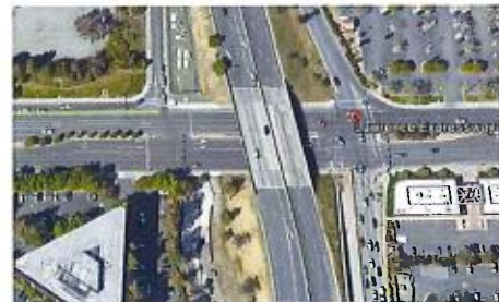
Lawrence Expressway ramp improvements
