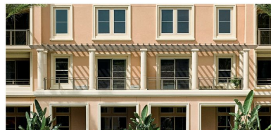
B. TRIM BAND PROFILE & ENHANCED PLASTER
